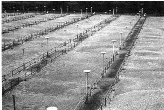
Figure 9.18 Scum covering the aeration basins at a wastewater treatment plant in Atlanta. (Courtesy of Mesut Sezgin.)
