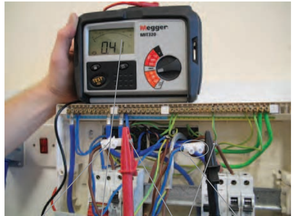
P2 joined to N1 Resistance 1/4 of that tested between N1 and P2 Test between joined ends P1 still joined to N2
