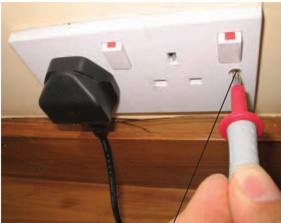
Screw fixings are earthed
