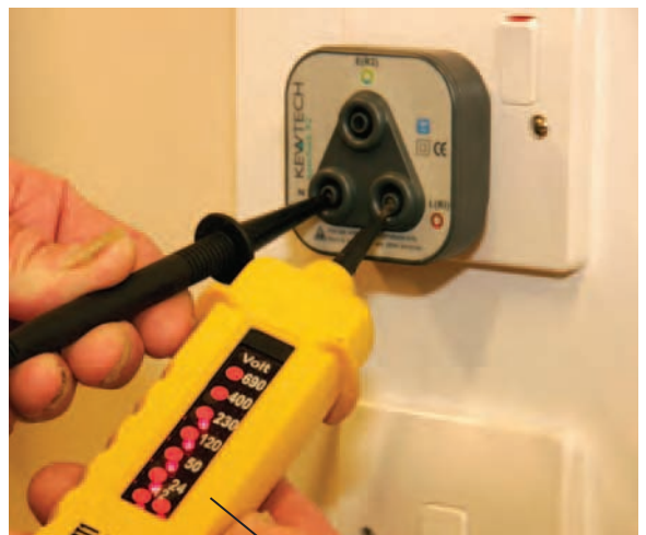
Voltage lights lit
