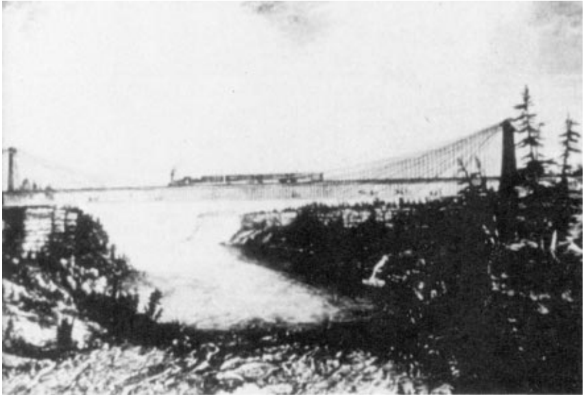
FIGURE 15.3 Niagara Falls Bridge.
