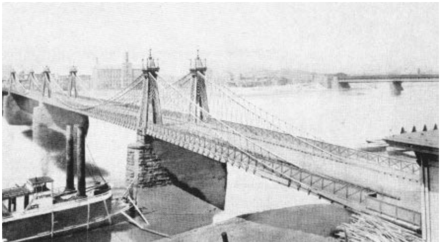
FIGURE 15.4 Old St. Clair Bridge, Pittsburgh.
