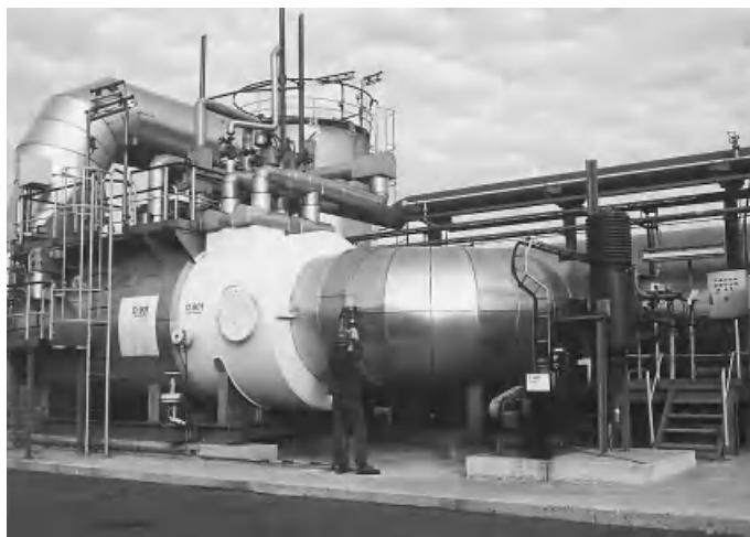
Fig. 8-2 Catalytic afterburning of the off-gases from a cyclohexanone plant (BASF, Antwerp)
