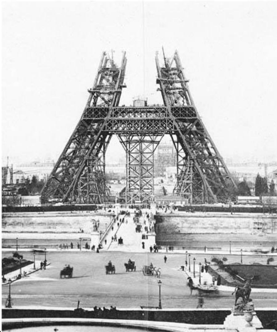
Eiffel's Tower under construction, Paris, 1888.
