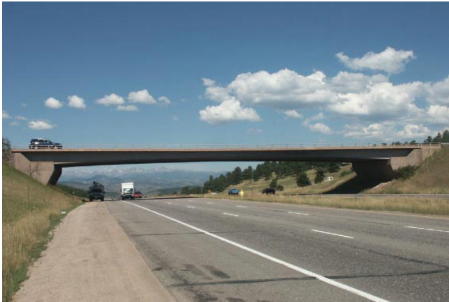
Exhibit 1.21 The Genesee Road (U.S. 40) Bridge over I-70 in Colorado is an elegant single span overcrossing with a slender appearance because the girder is in shadow and sloping lines on the abutment that invites the flow of traffic. It also provides a framework for an observer's first view of the Rocky Mountains. (Photo courtesy of Colorado DOT.)
