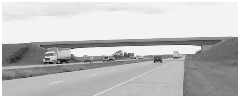
Fig. 3.27 Anchored end span bridge over I-39 located in north-central Illinois.
