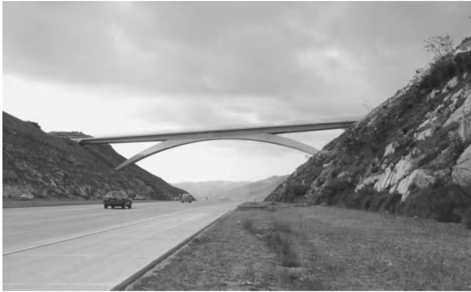
Fig. 3.15 Well-proportioned concrete arch, West Lilac Road overpass, I-15. (Permission granted by California DOT.)
