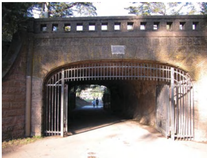
Exhibit 1.7 The Alvord Lake Bridge in San Francisco's Golden Gate Park was built in 1889 by Ernest Ransome. This reinforced concrete arch bridge is believed to be the oldest in the United States using steel reinforcing bars. It survived the 1906 San Francisco earthquake and several subsequent tremblers without damage and continues in service today. ( sanfranciscodays.com .)
