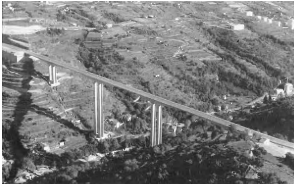
Fig. 3.6 Magnan Viaduct near Nizza, France (Muller, 1991). (From Bridge Aesthetics Around the World , copyright © 1991 by the Transportation Research Board, National Research Council, Washington, DC. Reprinted with permission.)
