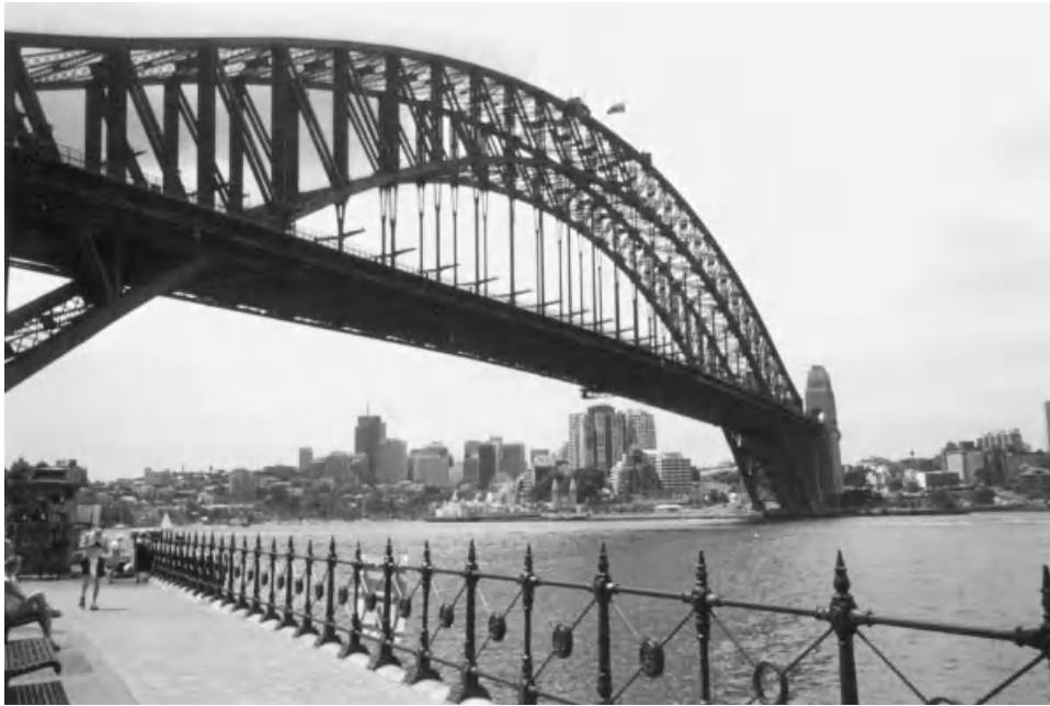
Fig. 4.9 Sydney Harbour Bridge.
