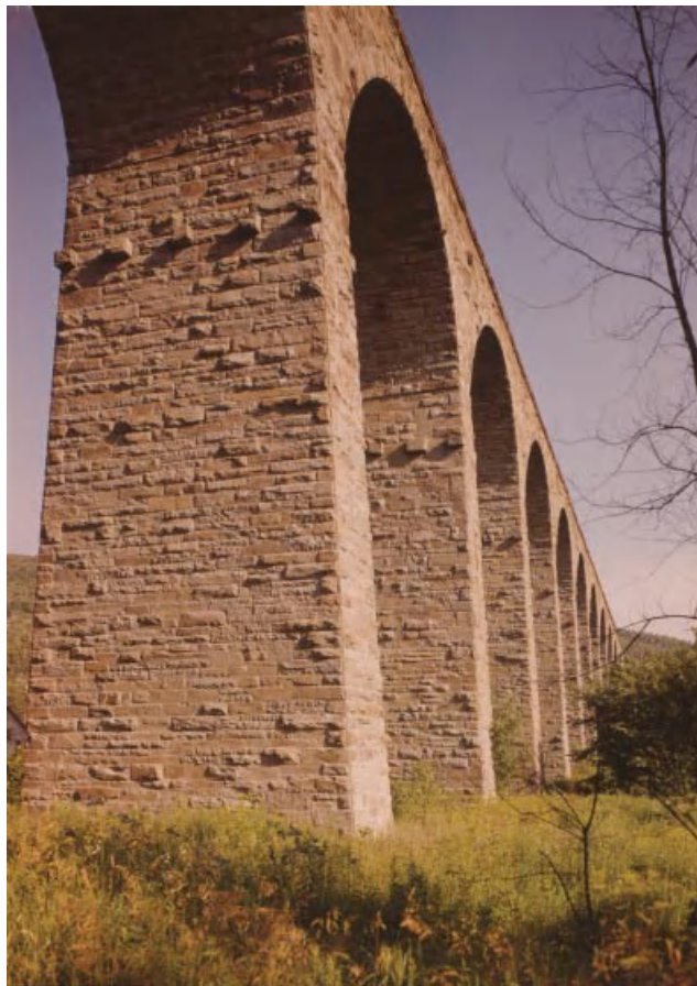
Exhibit 1.2 The Starrucca Viaduct near Lanesboro, Pennsylvania, was built in 1848 by the Erie Railway. At the time of its construction, it was the largest stone arch rail viaduct in the United States. The bridge has been in continual use for more than 160 years and still carries two tracks of the New York, Susquehanna and Western Railway. (HAER PA-6-17, photo by Jack E. Boucher, 1971.)
