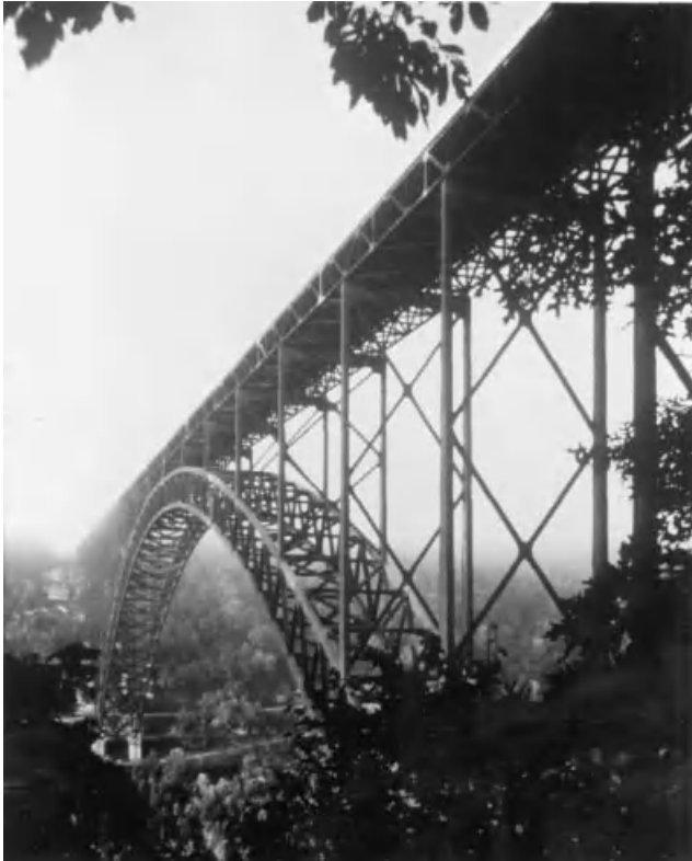
Fig. 1.13 New River Gorge Bridge. (Photo by Terry Clark Photography, courtesy of West Virginia Department of Transportation.)
