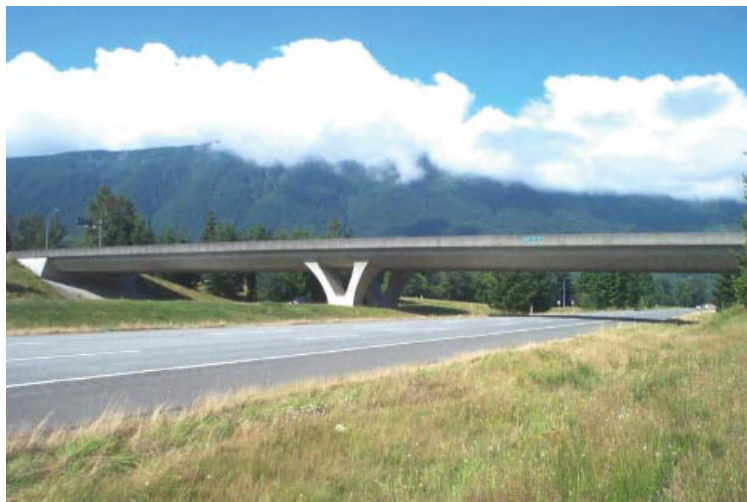
Exhibit 1.20 The 436th Avenue SE Undercrossing of I-90, King County, Washington, by increasing the mass of the central pier provides a focal point that successfully directs attention away from the split composition effect of the two-span layout and duality is resolved. (Photo courtesy of Washington State DOT.)
