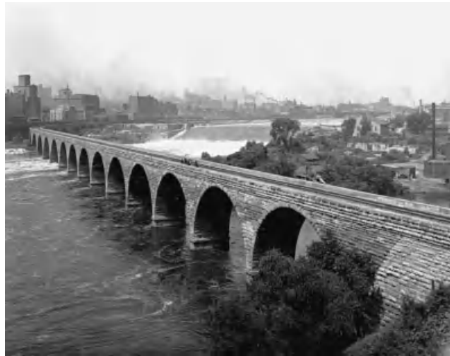
Fig. 1.1 James J. Hill Stone Arch Bridge, Minneapolis, Minnesota. (Hibbard Photo, Minnesota Historical Society, July 1905.)
