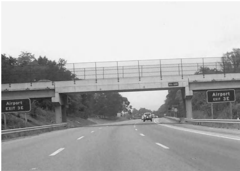
Fig. 3.21 Concrete barrier wall and short-span overpass without shadow: girders look deeper.
