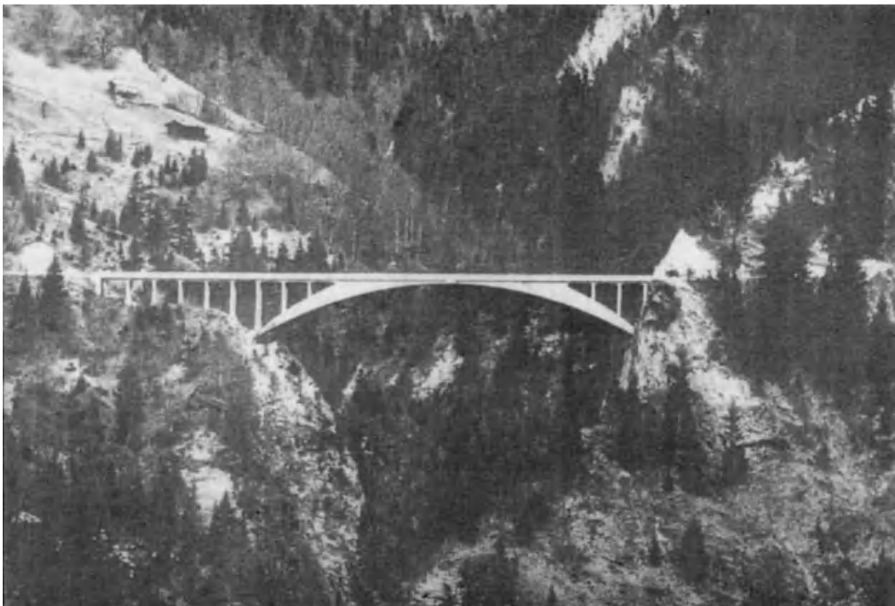
Fig. 4.2 General view of Salginatobel Bridge. [From Troitsky (1994). Reprinted with permission of John Wiley & Sons, Inc.]
