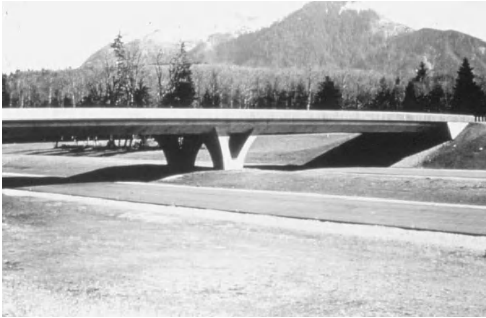
Fig. 3.23 436th Avenue SE Undercrossing, I-90, King County, Washington. (Photo courtesy of Washington State DOT.)
