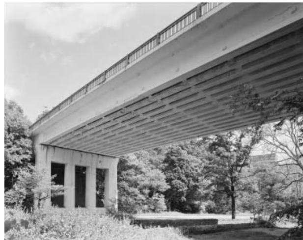
Exhibit 1.10 The Walnut Lane Bridge spanning Lincoln Drive and Monoshone Creek, Philadelphia, Pennsylvania, was designed by Gustave Magnel and constructed in 1949–1950. This bridge was the first prestressed concrete beam bridge built in the United States. It provided the impetus for the development of methods for design and construction of this type structure in the United States. (A. Pierce Bounds, 1988, HAER PA-125-5.)
