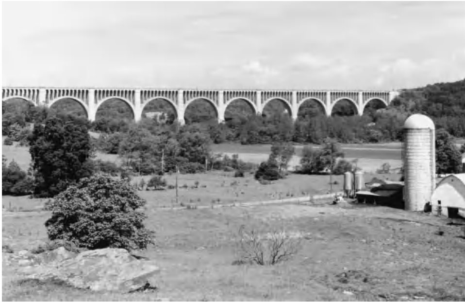
Fig. 3.17 Tunkhannock Viaduct near Nicholson, Pennsylvania, designed by A. Burton Cohen. (Jet Lowe, HAER Collection, Historic American Engineering Record.)
