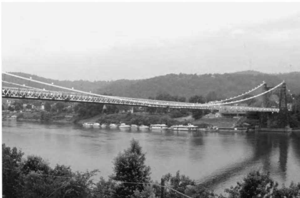
Fig. 1.11 Wheeling Suspension Bridge. (Photo by John Brunell, courtesy of West Virginia Department of Transportation.)
