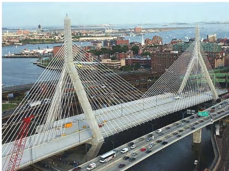
Exhibit 1.16 The Leonard P. Zakim Bunker Hill Memorial Bridge was designed by Christian Menn, completed in 2002, and spans the Charles River at Boston, MA. The towering bridge contrasts with the skyline of the city. It has become an icon and nearly as identifiable with Boston as the Eiffel Tower is to Paris. ( leonardpzakimbunkerhillbridge.org .)
