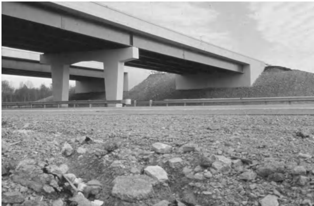
Fig. 3.35 Hammerhead piers. (Photo courtesy of Tennessee DOT—Geo. Hornal, photographer.)
