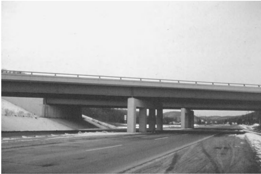
Fig. 3.36 Multiple-column bents. (Photo courtesy of Tennessee DOT—Geo. Hornal, photographer.)
