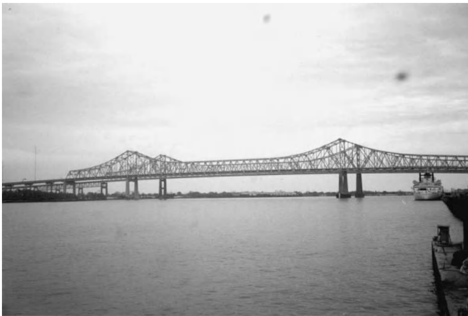
Fig. 4.6 Greater New Orleans Through-Truss Bridge. (Photo courtesy of Amy Kohls, 1996.)
