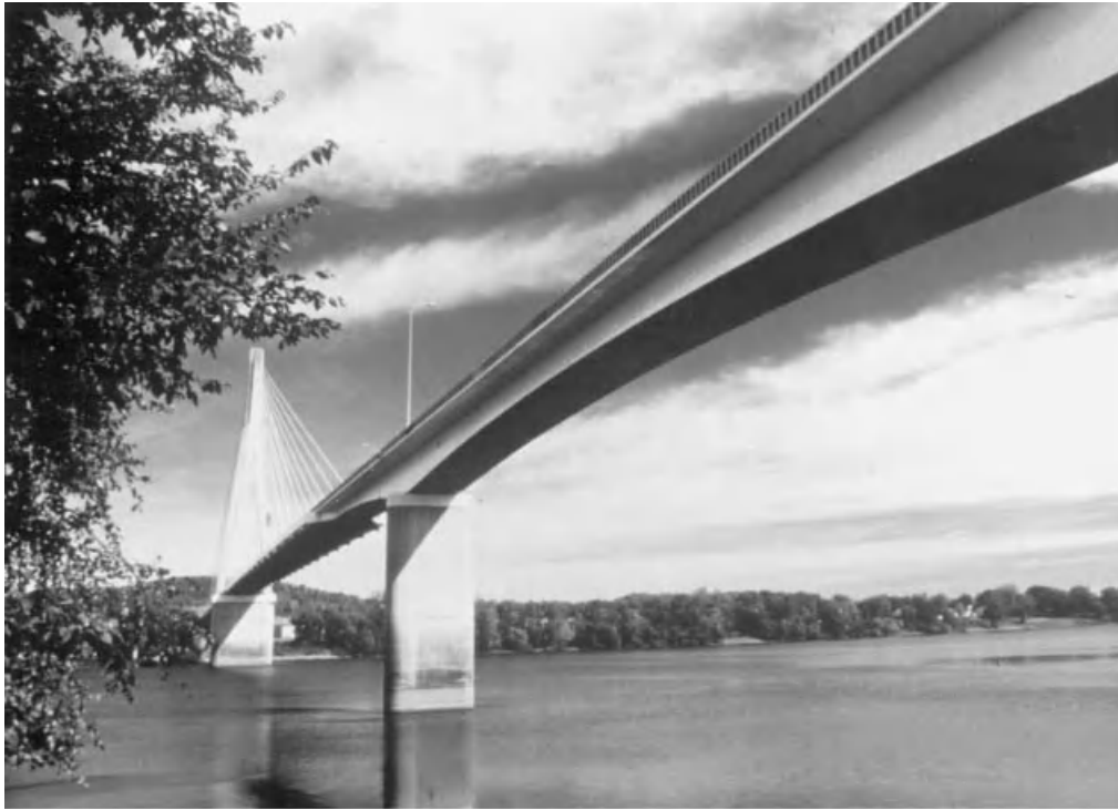
Fig. 3.18 East Huntington Bridge in Huntington, West Virginia. (Photo by David Bowen, courtesy of West Virginia DOT.)
