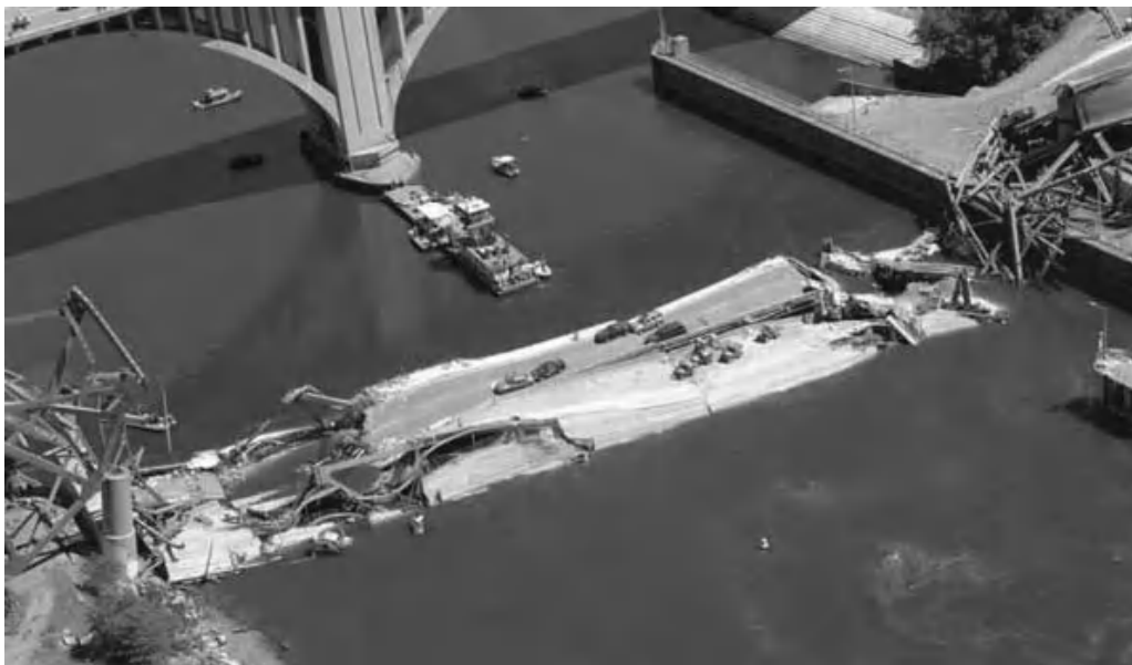
Fig. 2.16 Collapsed bridge center section, looking southeast (NTSB, 2008).
