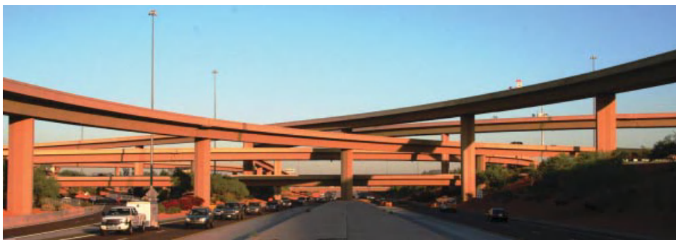
Exhibit 1.23 The I-17/101 Interchange in Phoenix, Arizona, has tapered textured piers supporting four levels of directional roadways. The piers and girders have different dimensions, but they all belong to the same family. (Photo courtesy of Arizona DOT.)
