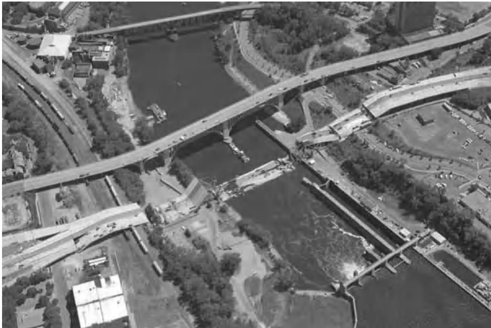
Fig. 2.12 Aerial view of I-35W Bridge after collapse (NTSB, 2008).
