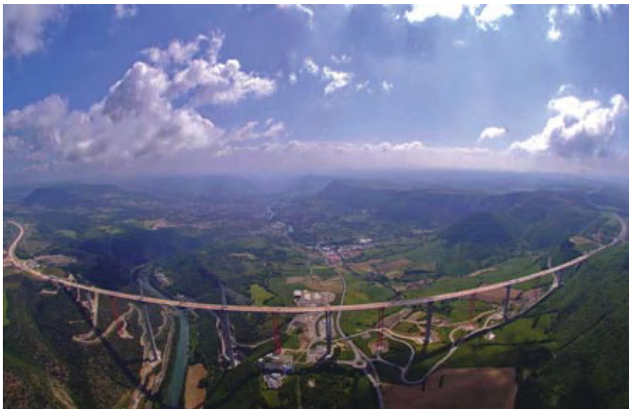
Exhibit 1.22 The Millau Viaduct spans the valley of the river Tarn near Millau in southern France. Completed in 2004, it has the tallest piers of any bridge in the world. The sweeping curve of the roadway provides stability as well as breathtaking views of the broad valley.
