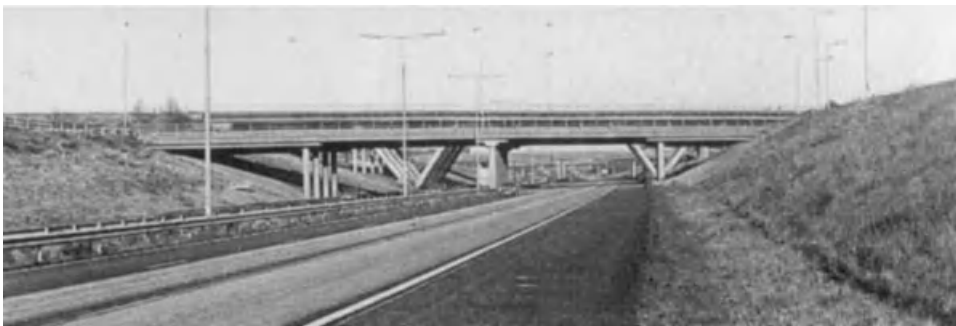
Fig. 3.14 Lack of harmony between adjacent bridges (Murray, 1991). (From Bridge Aesthetics around the World , copyright © 1991 by the Transportation Research Board, National Research Council, Washington, DC. Reprinted with permission.)
