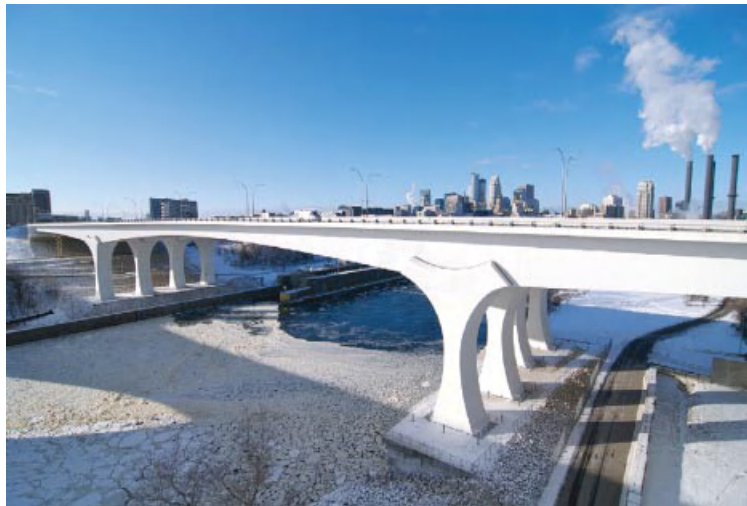
Exhibit 1.19 The I-35W St. Anthony Falls Bridge over the Mississippi River in Minneapolis, Minnesota, built in 2008 replaced the I-35W Bridge that collapsed in 2007 (see Section 2.2.7 and compare with Figure 2.14). The brightly lit girder face and sculpted piers contrast with the shadows cast by the deck overhang and the tops of the piers, accentuating the flow of the structure.
