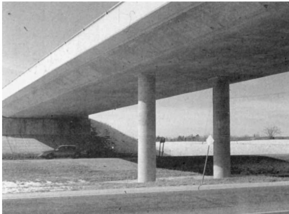
Fig. 4.8 Cast-in-place posttensioned voided slab bridge (Dorton, 1991). (From Bridge Aesthetics around the World , copyright © 1991 by the Transportation Research Board, National Research Council, Washington, DC. Reprinted with permission.)
