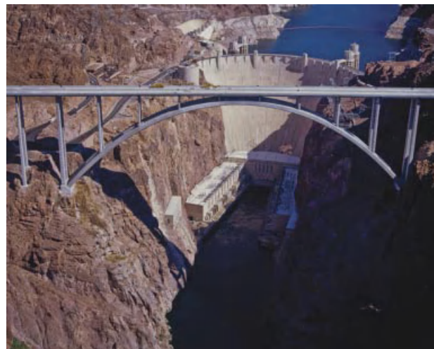
Exhibit 1.11 The Hoover Dam Bypass Bridge was completed in October, 2010, and was the first concrete-steel composite arch bridge (concrete for the arch and columns and steel for the roadway deck) built in the United States. The function of the bypass and bridge was to improve travel times, replace the dangerous approach roadway, and reduce the possibility of an attack or accident at the dam site. ( www.hooverdambypass.org/Const_PhotoAlbum.htm .)
