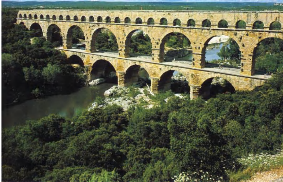
Exhibit 1.1 The Pont du Gard Aqueduct, Nîmes, France, was built by Romans 40–60 A.D. The lower arches were widened in 1743 to accommodate a road bridge.
