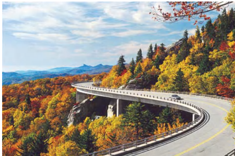
Exhibit 1.14 The Blue Ridge Parkway (Linn Cove) Viaduct, Grandfather Mountain, North Carolina, was built from the top down to protect the environment of Grandfather Mountain. This precast concrete segmental bridge was designed to blend in with the rugged environment.
