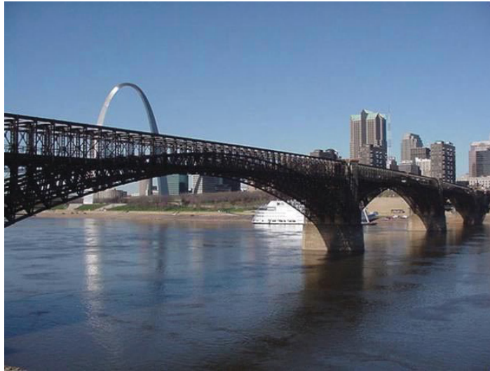
Exhibit 1.6 The Eads Bridge spanning the Mississippi River at Saint Louis, Missouri, was built 1867–1874 by James Buchanan Eads. The triple span, tubular metallic, arch construction required precise quality control and deep caissons to achieve its engineering and aesthetics success.
