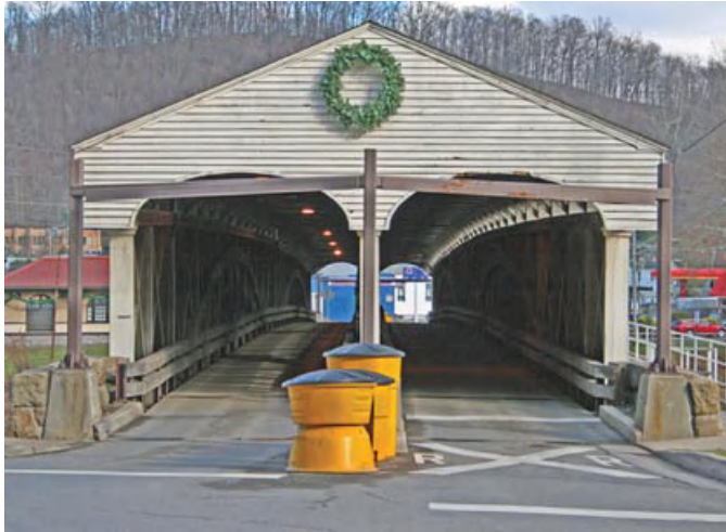
Exhibit 1.3 The Philippi Covered Bridge across the Tygart River Valley near Philippi, West Virginia, was built in 1852. It was used by armies of both the North and the South in the Civil War. In 1934 the bridge was strengthened and is today a part of U.S. 250. It is reportedly the only remaining two-lane “double barrel” covered bridge.
