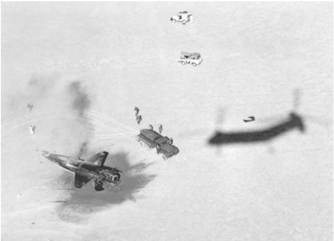
Aftermath of Jack McKay's rollover accident on 9 November 1962. X-15 no. 2 is pointing nearly back along its flight path, and the shadow of the H-21 helicopter is on the right. The H-21 used its downwash to protect McKay from fumes when he was still trapped upside down in the cockpit. Courtesy of the Dryden Flight Research Center.
