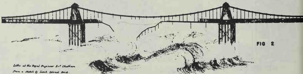
SKETCH Showing the appearance of the 3 rd Span after it gave way.
