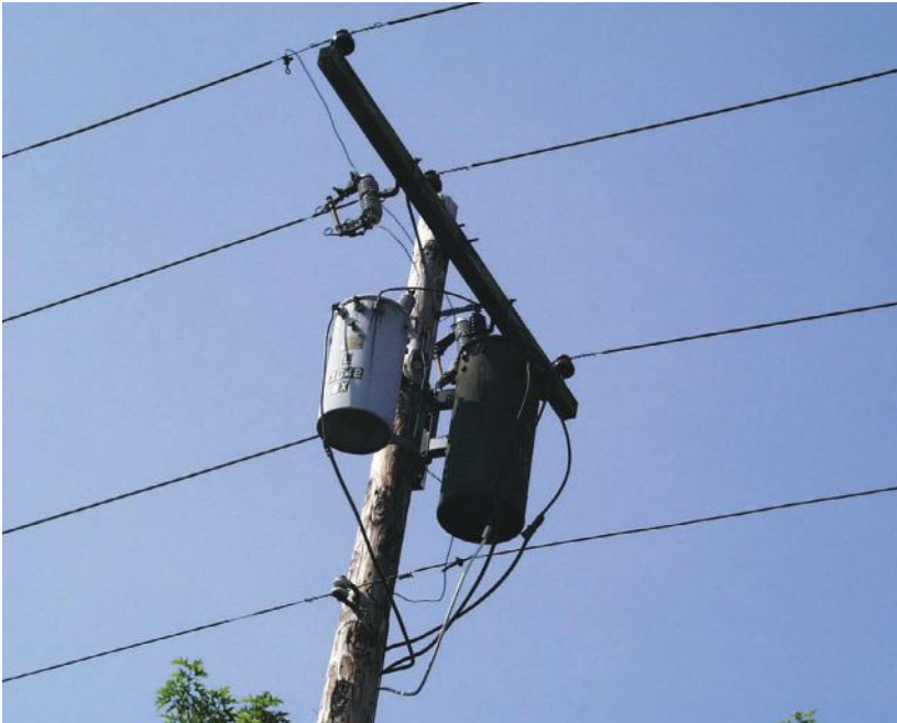
FIGURE 8.8 Single circuit distribution line.
