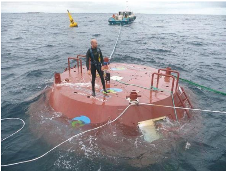
FIGURE 6.77 Buoyant actuator during the installation. (Courtesy of Carnegie Wave Energy through Wikipedia.)
