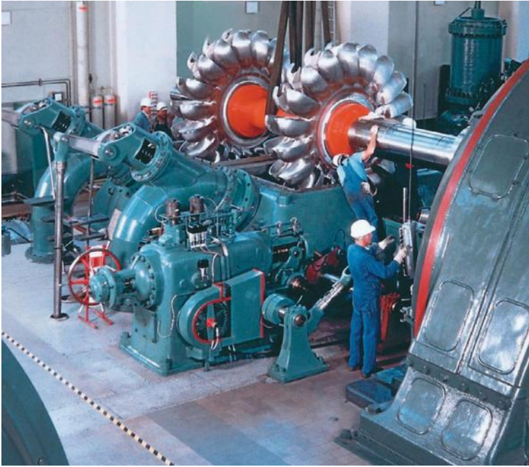
FIGURE 4.9 Pelton turbine being installed. (Courtesy of Siemens Hydro Power through Wikipedia.)
