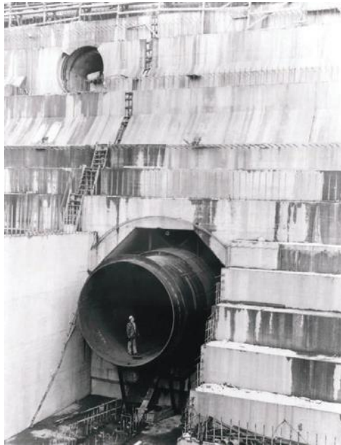
FIGURE 4.4 Penstock of Grand Coulee Dam. (Image courtesy of U.S. Bureau of Reclamation, Washington, DC.)
