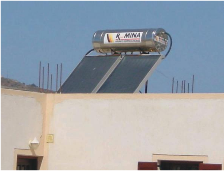
FIGURE 6.5 Passive thermosiphon hot water solar system.
