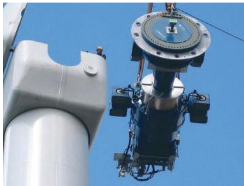
FIGURE 6.58 Lifting of gearbox and brakes of HAWT. (Courtesy of Paul Anderson through Wikipedia.)
