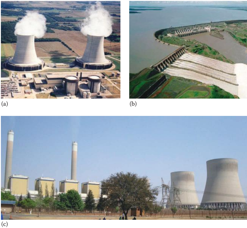
FIGURE 2.3 Power plants (a) nuclear, (b) hydro, (c) thermal.
