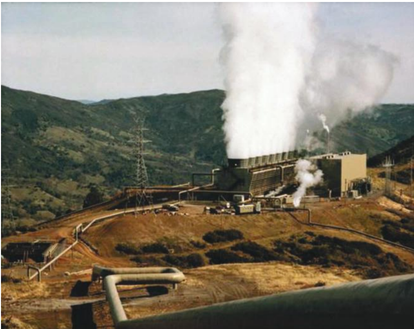
FIGURE 6.93 The Geysers in northern California—the first geothermal power plant in the United States.
