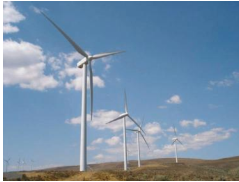
FIGURE 6.57 Horizontal axis wind turbines.
