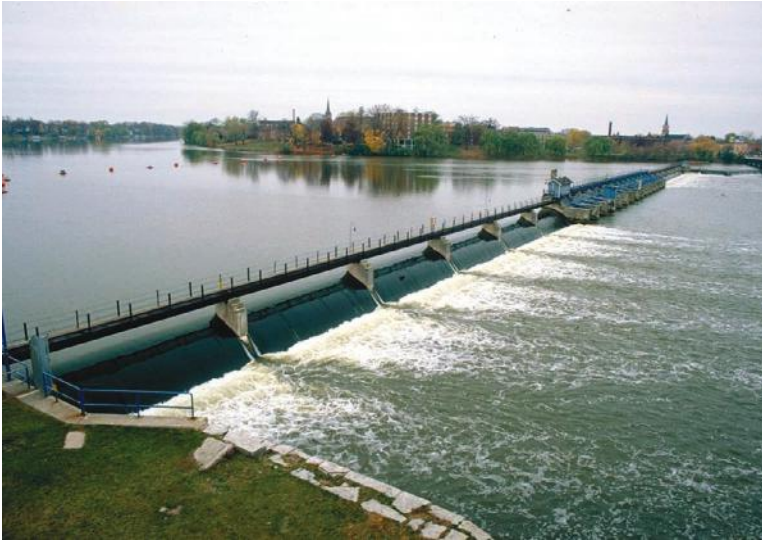
FIGURE 4.2 Fox River diversion hydroelectric power plant, Wisconsin. (Image courtesy of U.S. Army Corps of Engineers, Louisville, KY.)
