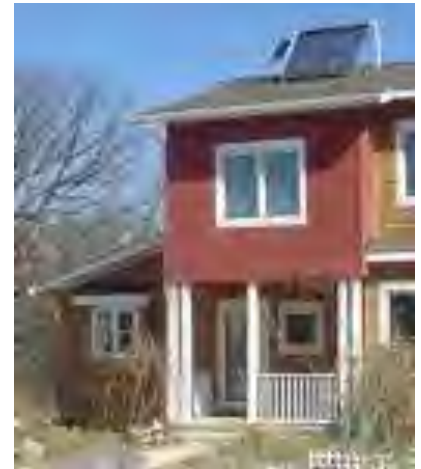
Figure 30.2. A solar water heater providing hot water for a family in Michigan. The system's pump is powered by the small photovoltaic panel on the left.
