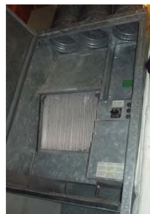
Figure E.11. The Heatkeeper's heat-exchanger.
