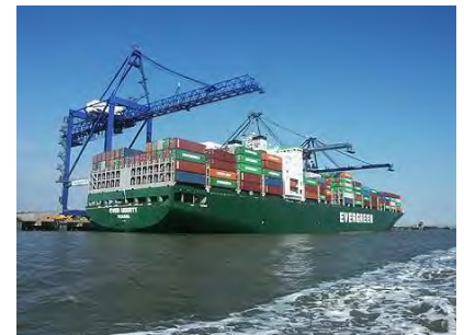
Figure 15.6. The container ship Ever Uberty at Thamesport Container Terminal. Photo by Ian Boyle www.simplonpc.co.uk .
