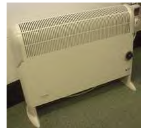
Figure 7.6. A big electric heater: 2 kW.
