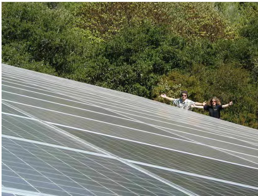
Figure 6.6. Two solar warriors enjoying their photovoltaic system, which powers their electric cars and home. The array of 120 panels ( 300\text{ W} each, 2.2\text{ m}^2 each) has an area of 268\text{ m}^2 , a peak output (allowing for losses in DC-to-AC conversion) of 30.5\text{ kW} , and an average output – in California, near Santa Cruz – of 5\text{ kW} ( 19\text{ W/m}^2 ). Photo kindly provided by Kenneth Adelman.
