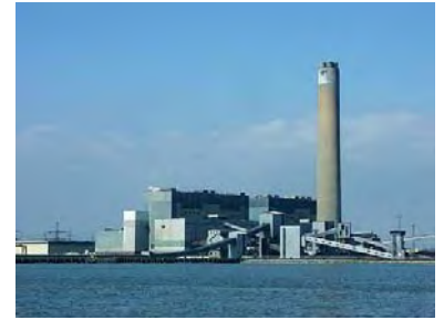
Figure 23.1. Coal being delivered to Kingsnorth power station (capacity 1940 MW) in 2005. Photos by Ian Boyle www.simplonpc.co.uk .
