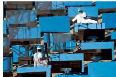
Figure 25.12. Two engineers assembling an eSolar concentrating power station using heliostats (mirrors that rotate and tip to follow the sun). esolar.com make medium-scale power stations: a 33 MW (peak) power unit on a 64 hectare site. That's 51 \text{ W/m}^2 peak, so I'd guess that in a typical desert location they would deliver about one quarter of that: 13 \text{ W/m}^2 .
