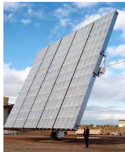
Figure 25.9. A 25 kW (peak) concentrator photovoltaic collector produced by Californian company Amonix. Its 225 \text{ m}^2 aperture contains 5760 Fresnel lenses with optical concentration \times 260 , each of which illuminates a 25%-efficient silicon cell. One such collector, in an appropriate desert location, generates 138 kWh per day – enough to cover the energy consumption of half an American. Note the human providing a scale. Photo by David Faiman.
