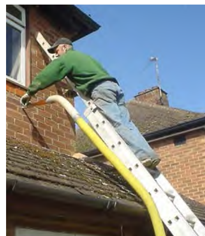
Figure 21.5. Cavity-wall insulation going in.
