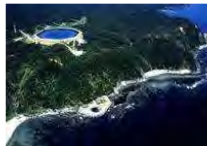
Figure 26.11. Okinawa pumped-storage power plant, whose lower reservoir is the ocean. Energy stored: 0.2 GWh. Photo by courtesy of J-Power. www.ieahydro.org .
