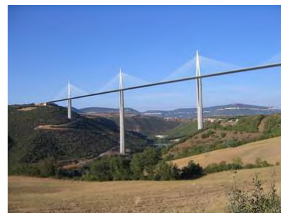
Figure H.7. Millau Viaduct in France, the highest bridge in the world. Steel and concrete, 2.5 km long and 353 m high.
