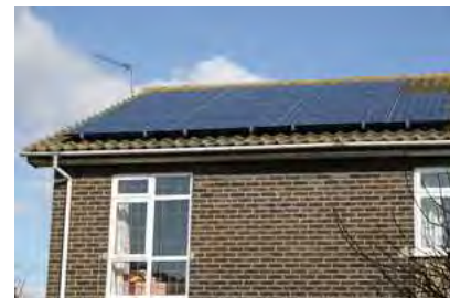
Figure 6.5. Solar photovoltaics: data from a 25\text{-m}^2 array in Cambridgeshire in 2006. The peak power delivered by this array is about 4\text{ kW} . The average, year-round, is 12\text{ kWh} per day. That's 20\text{ W} per square metre of panel.
