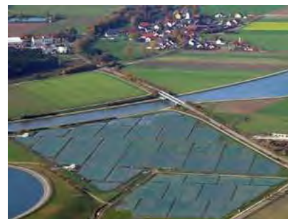
Figure 6.7. A solar photovoltaic farm: the 6.3 MW (peak) Solarpark in Mühlhausen, Bavaria. Its average power per unit land area is expected to be about 5 \text{ W/m}^2 . Photo by SunPower.
