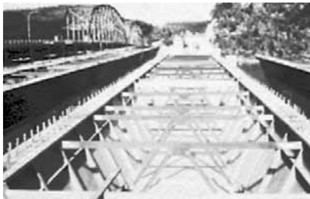
FIGURE 51.1 Composite box girders, Hawkesbury River Bridge, Australia.
