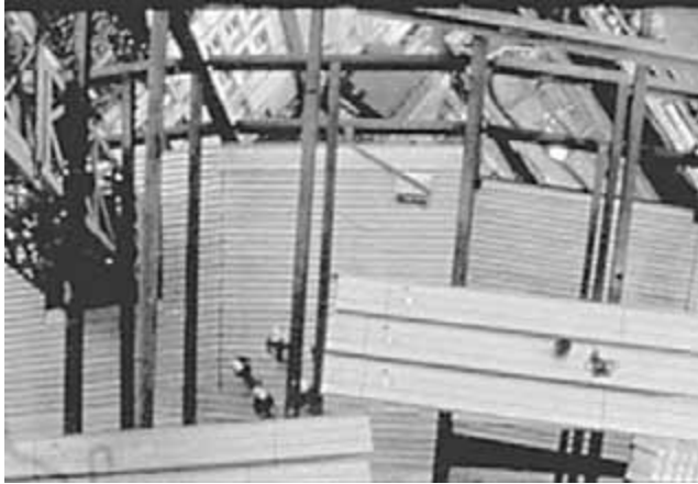
FIGURE 51.2 Composite steel–concrete floors, Grosvenor Place, Sydney.
