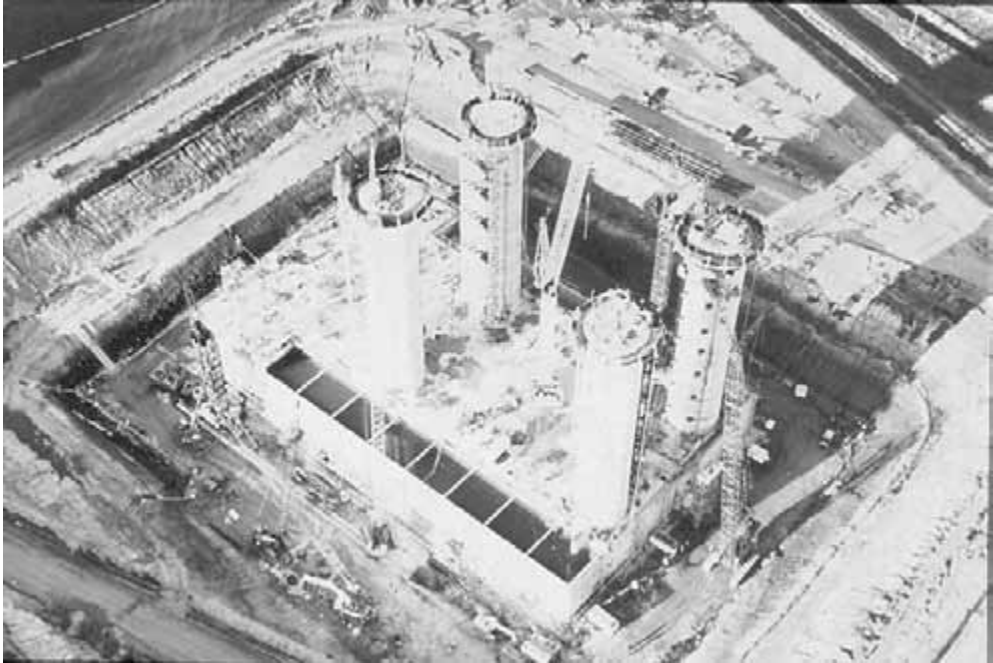
FIGURE 42.2 Wandoo platform under construction in western Australia.
