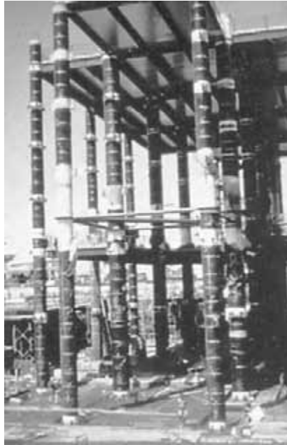
FIGURE 42.4 Steel tube columns at Market City, Australia.
