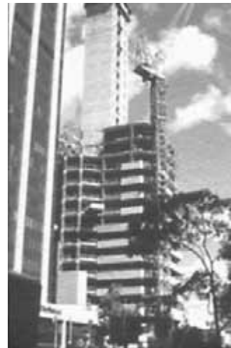
FIGURE 51.5 Composite construction, Forrest Place, Perth.
