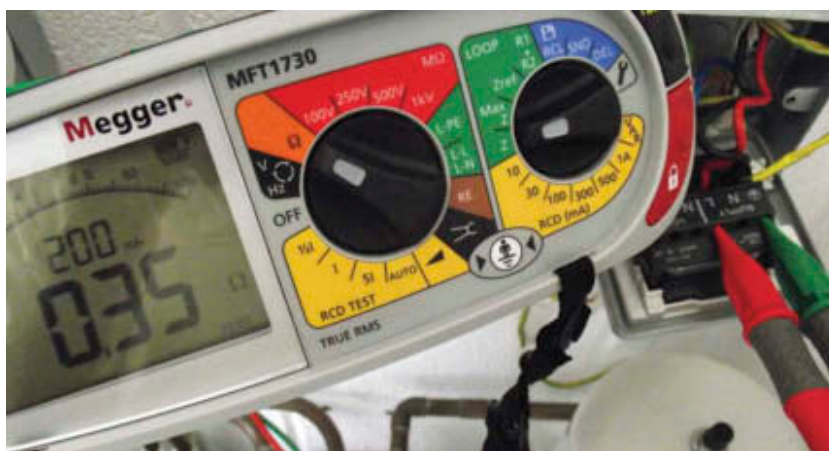
Figure 4.55 Test between line and earth R_1 + R_2
