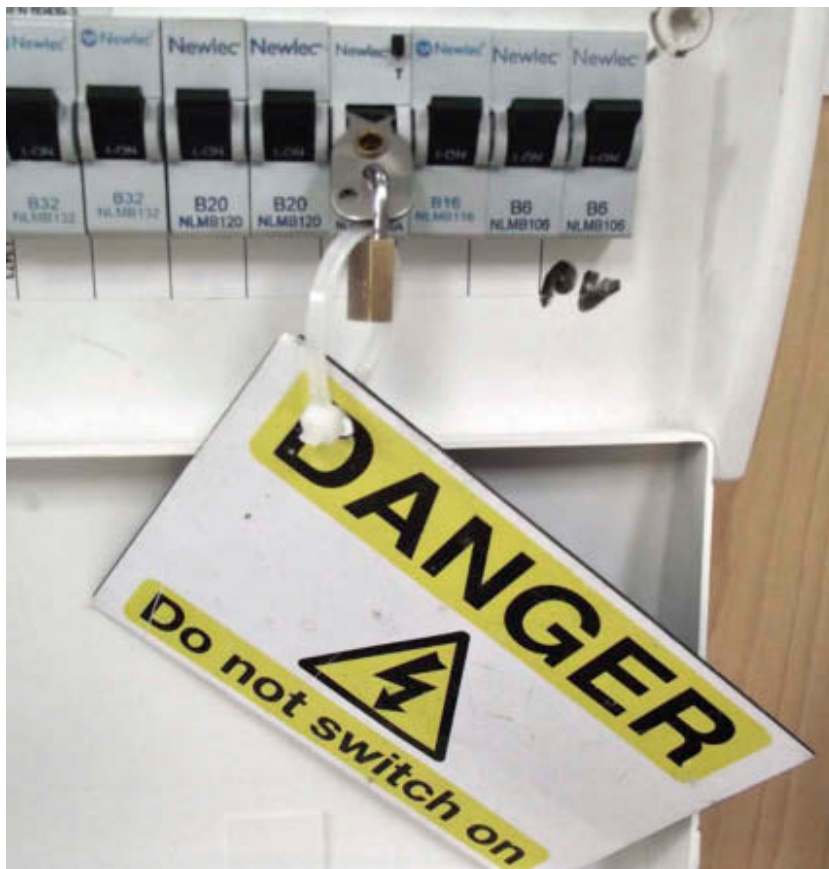
Figure 4.8 Locked off
