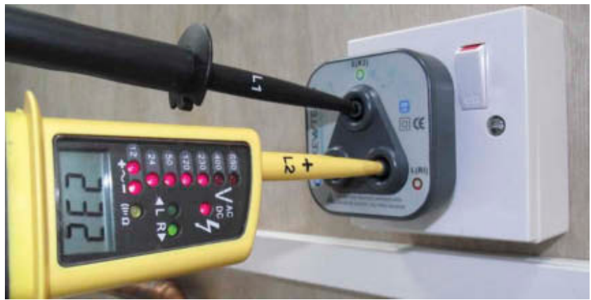
Figure 4.7a Test line to earth
