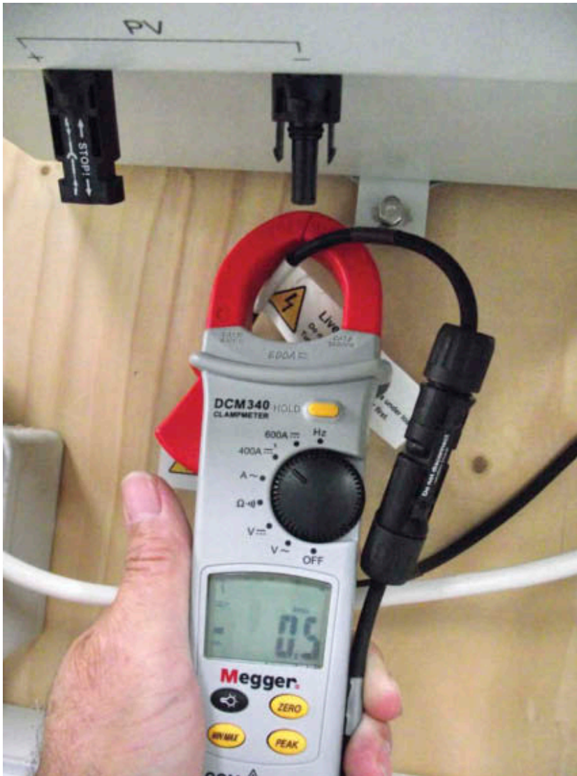
Figure 10.10 Current measurement using clamp meter
