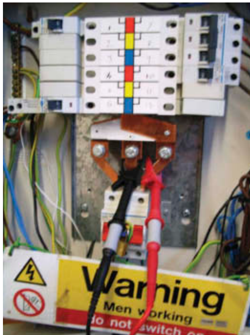
Figure 4.51a Test L2 to L3
