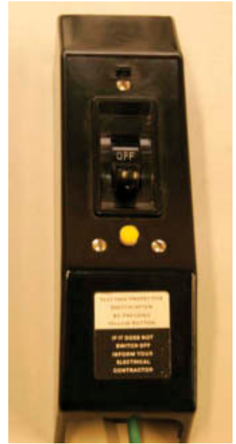
Figure 5.29 Voltage operated RCD
