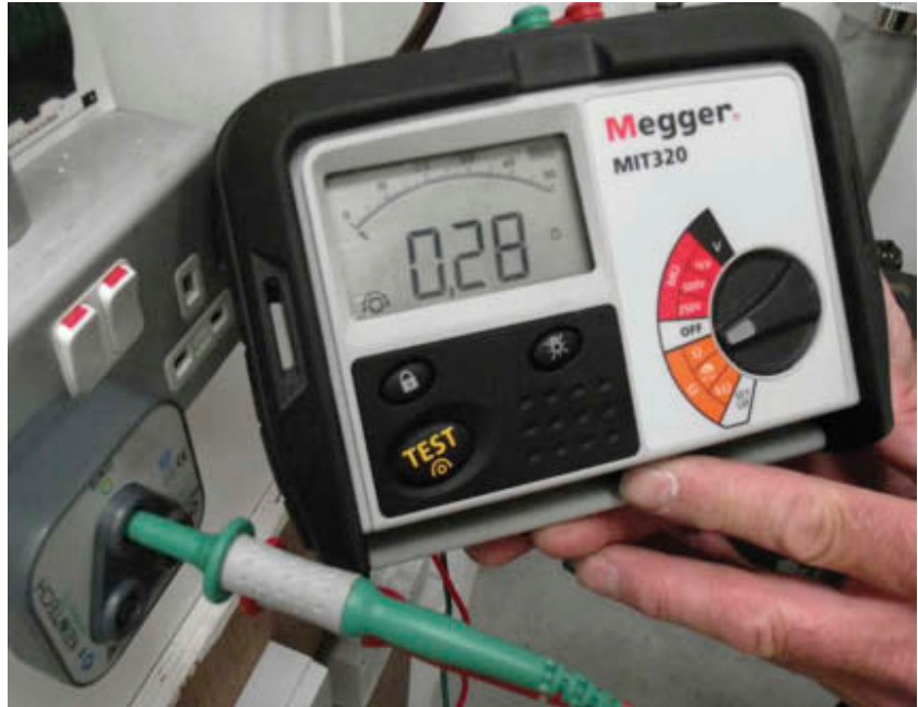
Figure 4.39 Test line to earth at each socket
