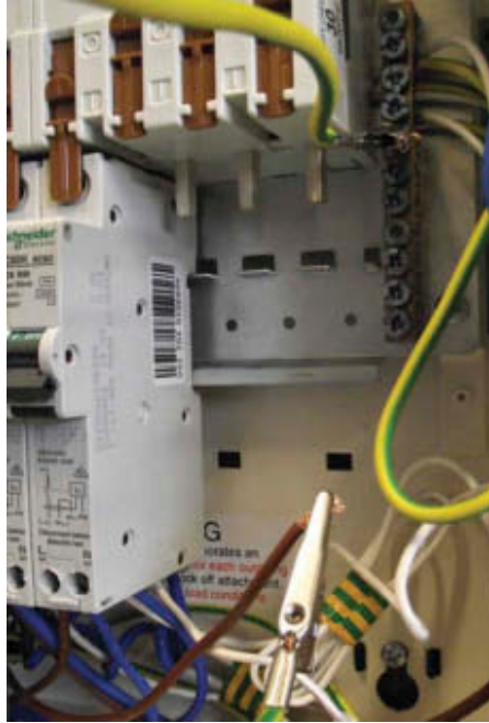
Figure 4.61 Line and earth terminal linked
