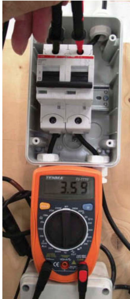
Figure 10.11 Current measurement using a multimeter
