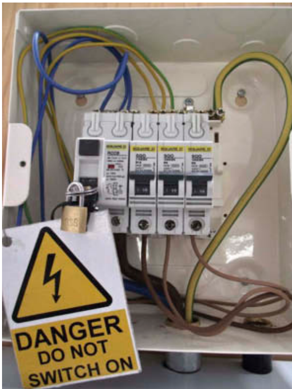
Figure 4.12 Isolate the supply
