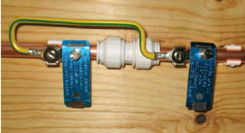
Figure 4.23 Fitting bonded across
