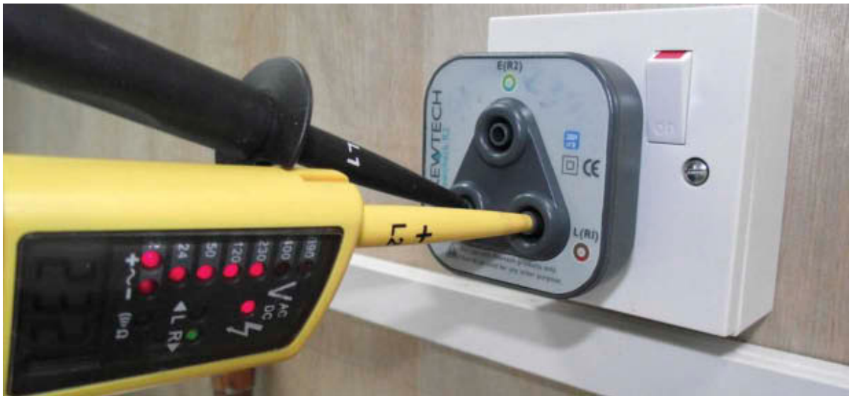
Figure 4.6 Test line to neutral
