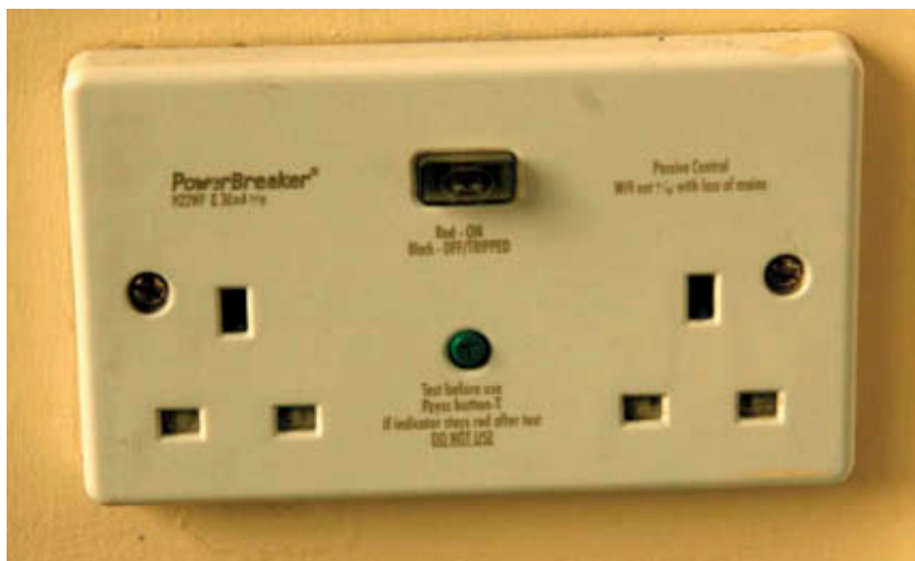
Figure 5.34 RCD socket outlet
