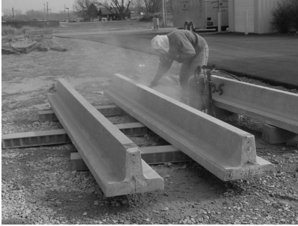
FIGURE 8.4 Surface preparations by sandblasting.
