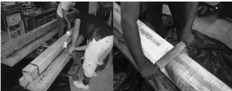
FIGURE 8.8 Applying resin to FRP with a paint roller (left) and clearing the air pockets with a wooden roller (right).
