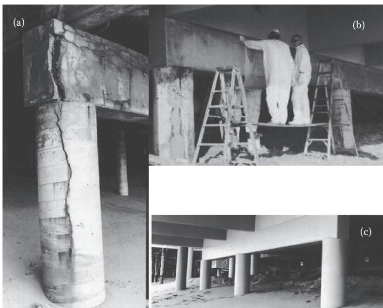
FIGURE 8.2 Damage caused by corrosion: (a) before repair, (b) after repair prior to strengthening, and (c) after strengthening. (Courtesy of Fyfe Inc.)
