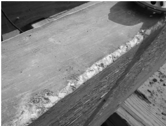
FIGURE 8.5 Rounded beam corners by grinding.
