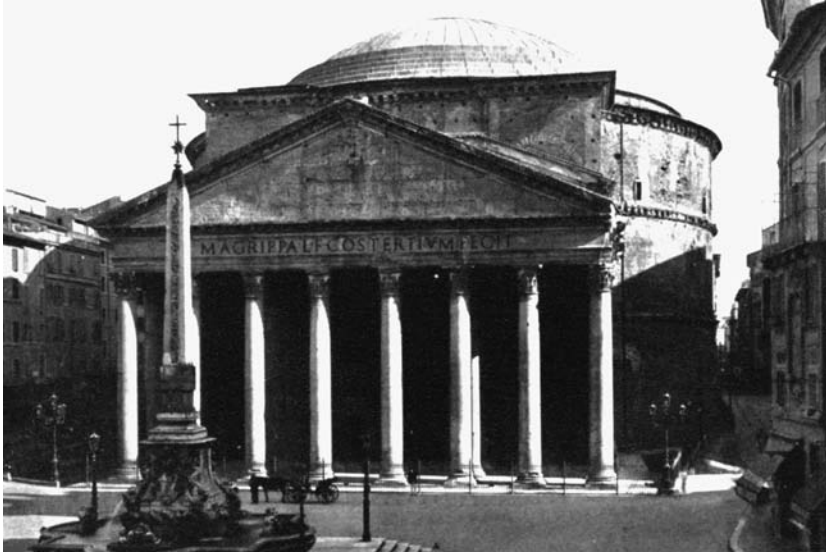
Figure 7.2 The Pantheon, Rome, built using pumice as lightweight aggregate in the concrete of the dome (2nd century AD).
