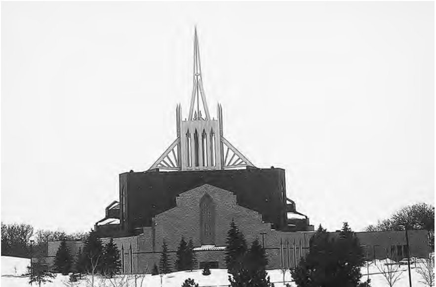
FIGURE 7.14. Exterior, Wooddale Church, Eden Prairie, Minn., 1990. Milo Thompson, architect. Photo by William P. Halgren.
