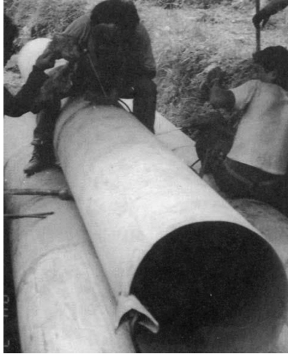
FIGURE 7.14 Site welding of penstock pipe.
