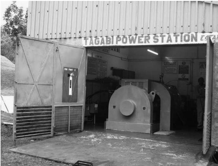
FIGURE 2.22 A powerhouse building of a 900-kW mini hydropower plant, Kenya.
