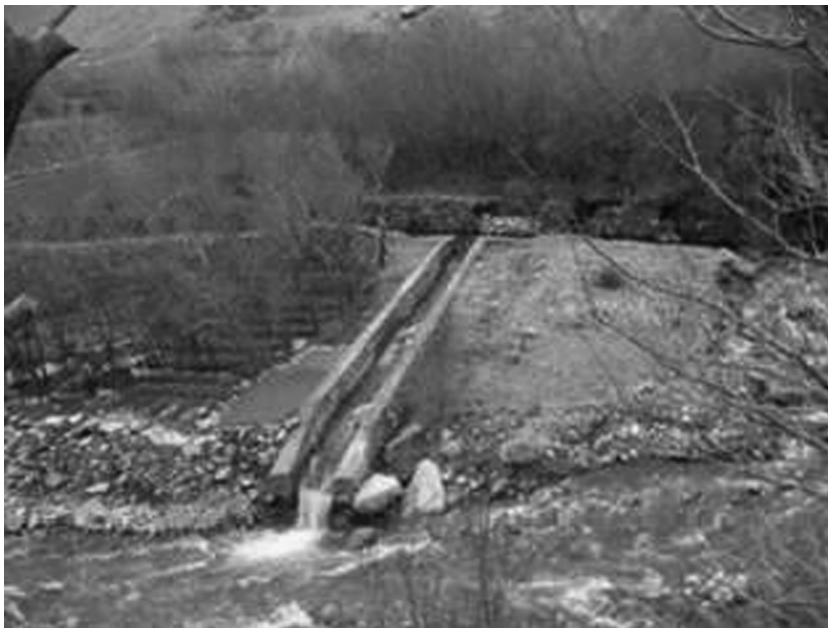
FIGURE 2.14 Spillway located along an irrigation canal, Afghanistan.
