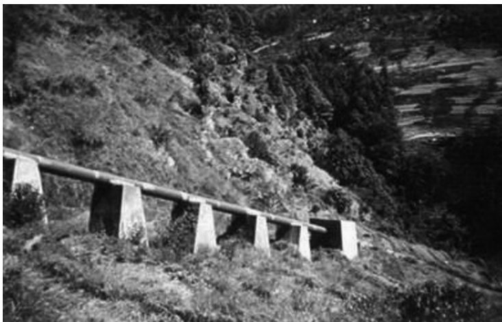
FIGURE 2.21 Masonry support piers used in a mini hydropower plant, Nepal.
