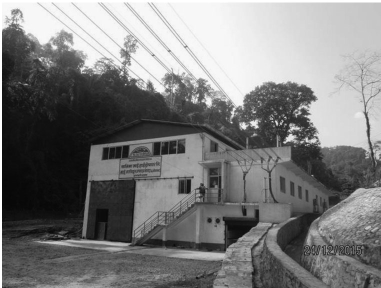
FIGURE 8.10 Powerhouse of Mai hydropower plant.
