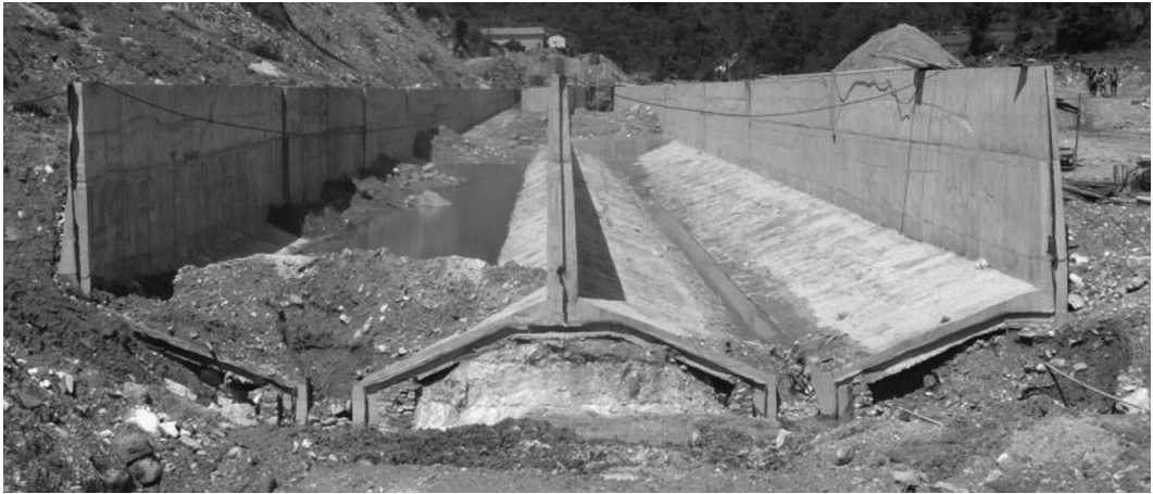
FIGURE 6.16 Settling basin main body during construction.
