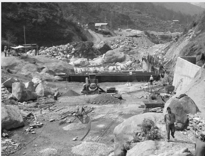
FIGURE 4.12 Boulder diversion weir under construction 2.5 MW Sun Koshi Hydropower Plant, Nepal.
