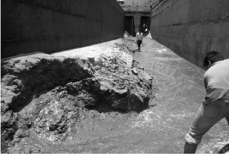
FIGURE 6.21 Sediments deposited in settling basin.
