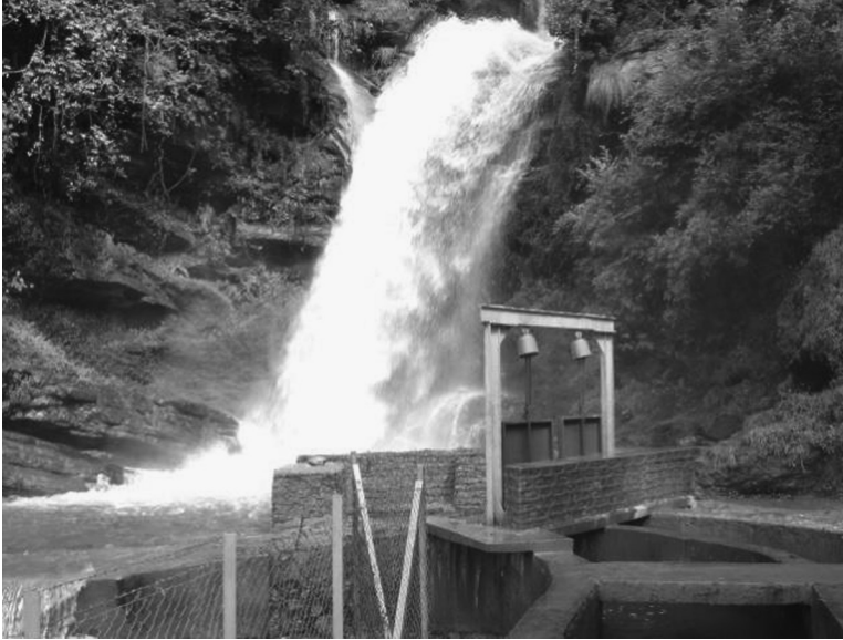
FIGURE 2.7 Typical side intake used in a small hydroelectric power plant, Nepal.
