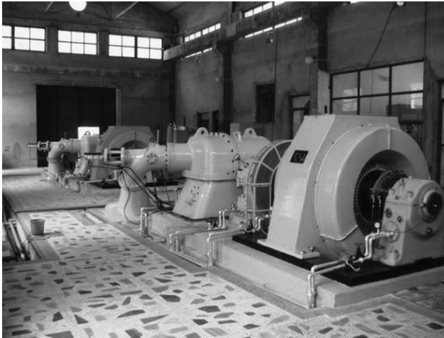
FIGURE 2.28 Turbine governor of a 2.5-MW small hydropower plant, Nepal.
