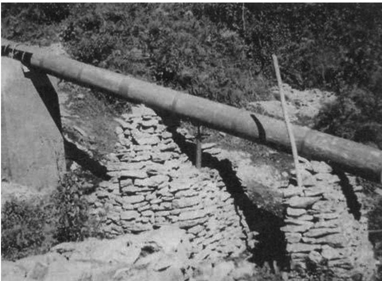
FIGURE 7.17 Temporary support for site welding work.
