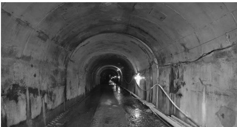
FIGURE 2.10 A 22-MW Mai hydropower plant's headrace tunnel near completion, Nepal.
