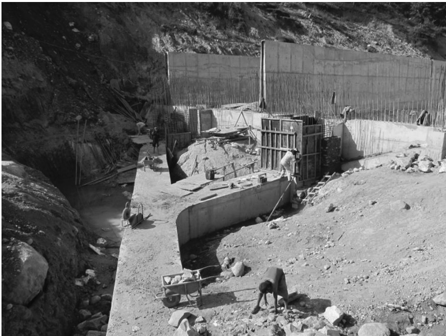
FIGURE 6.17 Flushing culvert and gates of settling basin (under construction).
