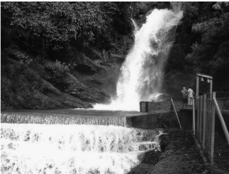
FIGURE 4.7 500-kW Jhankre mini hydropower plant, Nepal, with a semipermanent gabion weir.
