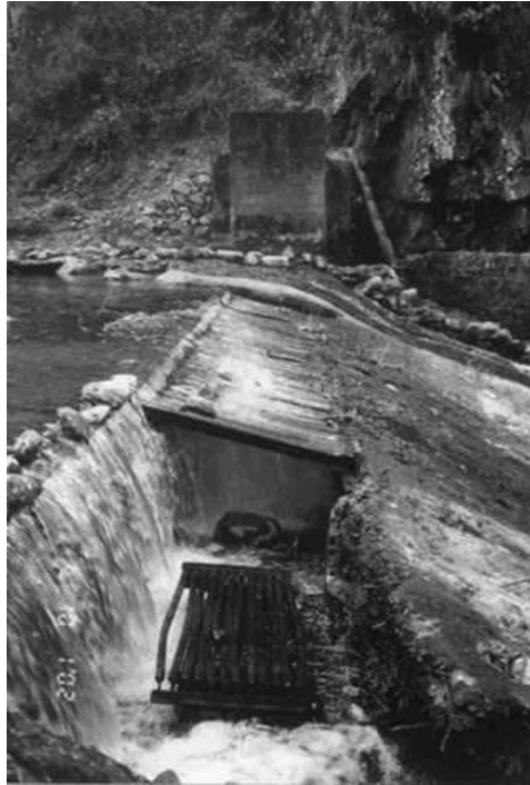
FIGURE 4.4 A typical bottom intake of a micro hydropower plant, Nepal.
