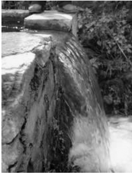
FIGURE 2.13 Spillway located at forebay wall in a micro hydropower plant, Afghanistan.
