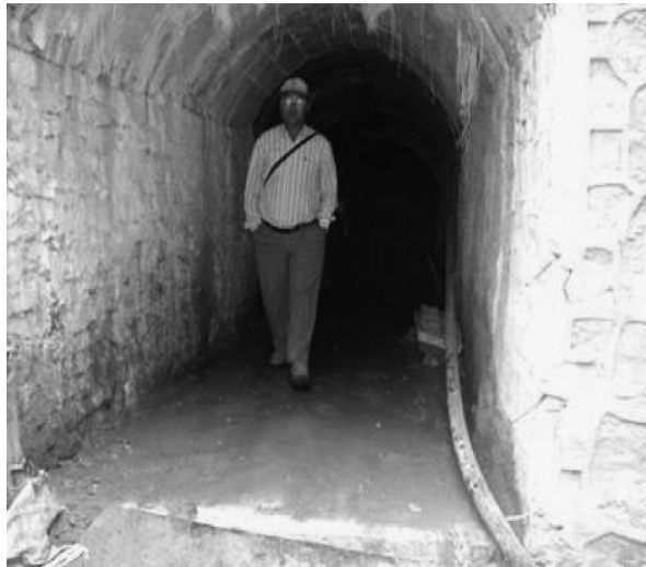
FIGURE 5.3 An under-construction headrace tunnel in a 3.0 MW Chaku hydropower plant, Nepal.
