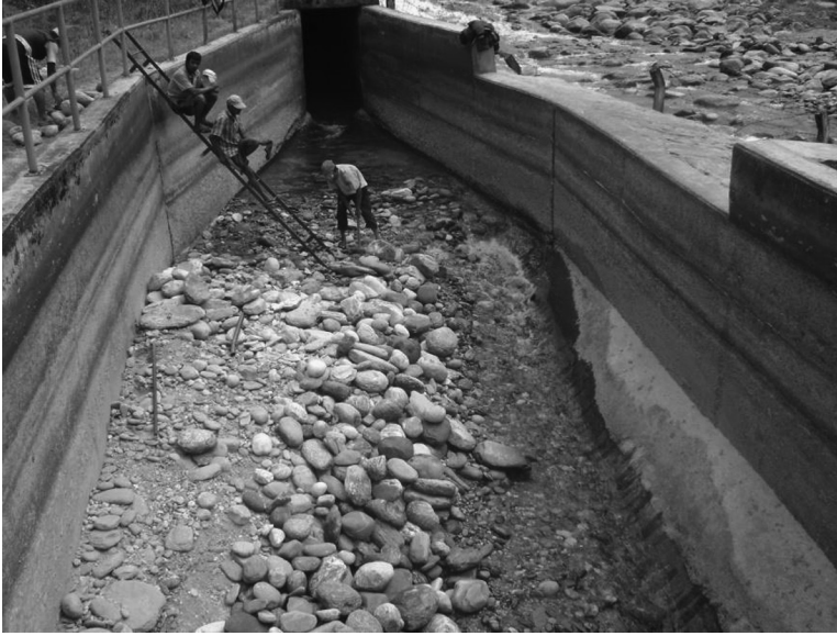
FIGURE 6.7 Large sediments deposited in the gravel trap.
