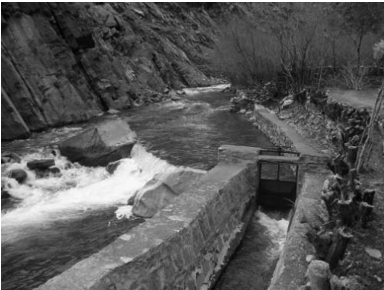
FIGURE 2.8 A frontal intake used in a micro hydropower plant, Afghanistan.
