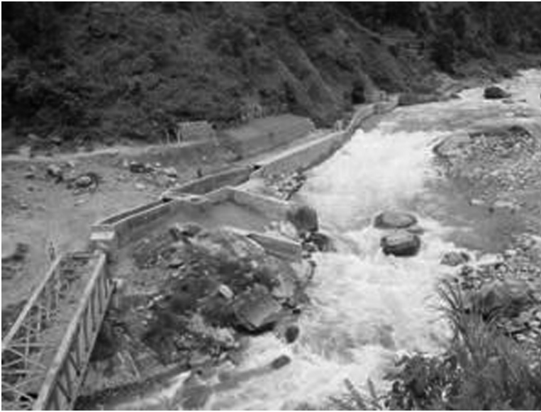
FIGURE 4.2 Side intake of 2.5-MW Sun Koshi Hydropower Plant, Nepal.
