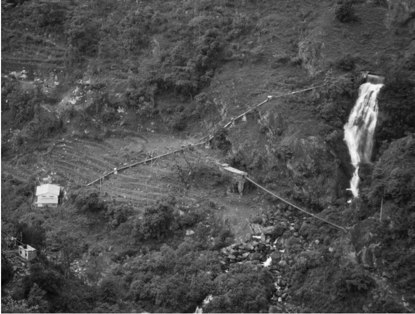
FIGURE 2.5 A 183-kW Syange (run-of-river) hydropower plant, Lamjung Nepal (notice that as this is a run-of-river plant, the excess water flows down the weir along the river and the penstock begins close to the intake).
