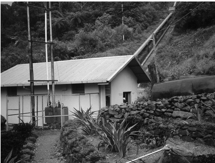
FIGURE 2.23 A powerhouse building for a micro hydropower plant, Indonesia.
