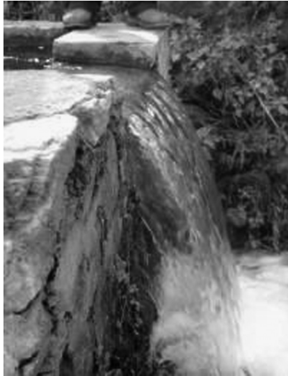
FIGURE 5.9 A spillway located at the forebay end wall.
