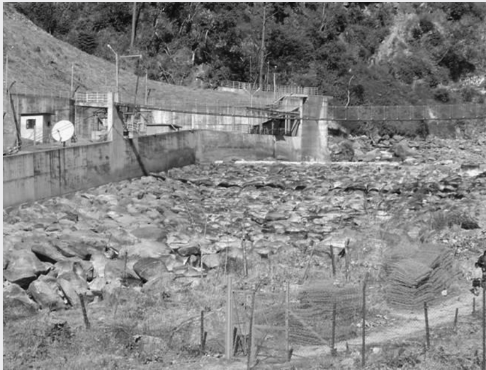
FIGURE 4.11 Boulder-lined, low-height diversion weir 60 MW Khimti, Nepal.
