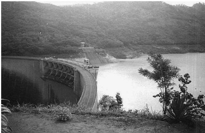
FIGURE 2.34 70-MW Victoria Dam in Sri Lanka.
