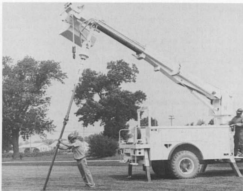
Figure C.3. Installation of helical anchor. (Courtesy of A. B. Chance Company, Centralia, Missouri, U.S.A.)
