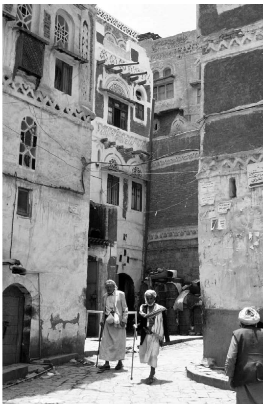
FIGURE 3. Old City. Yemen was until recently still impervious to blind development. Sana'a, 1993. Photo by author.
