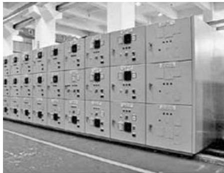
FIGURE 7.1 Medium-voltage switchgear
