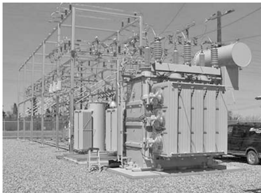
FIGURE 5.7 Conservator tank design
