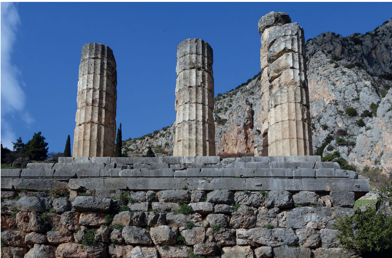
Figure 77 Remains of the Temple of Apollo, Delphi, looking West, limestone ( Profitis Ilias ) foundation blocks and marble columns, 4th century BCE. © Archaeological Site of Delphi, Hellenic Ministry of Culture and Sports, Ephorate of Antiquities of Phocis – Archaeological Receipts Fund. Photo courtesy of Dr. Steven Zucker
