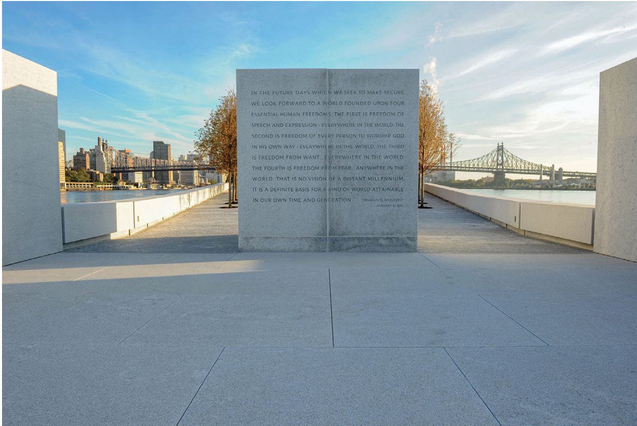
Figure 87 Louis I. Kahn, Franklin D. Roosevelt Four Freedoms State Park, New York, granite from Mount Airy, NC, designed 1973 and completed 2010–2012. Photo: Diane Bondereff
