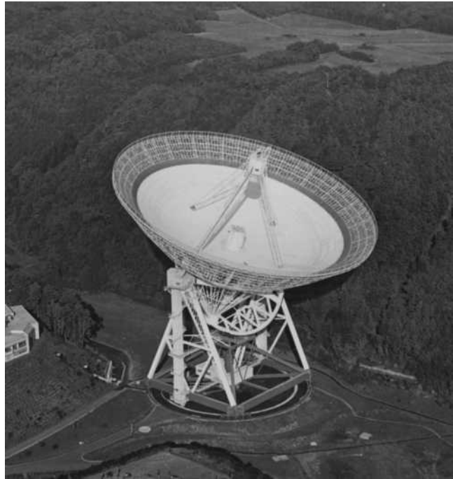
The 328-ft-diameter (100-m) radio telescope operated by the Max Planck Institut für Radioastronomie at Effelsberg, Germany. (Max Planck Institut für Radioastronomie)
