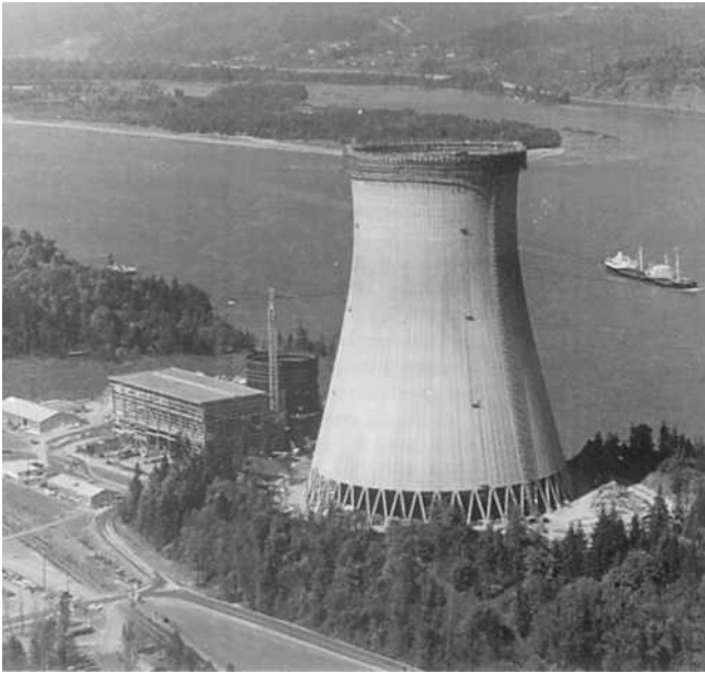
Counterflow natural-draft cooling tower at Trojan Power Plant in Spokane, Washington. ( Research-Cottrell )
