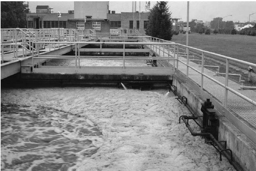
Figure 17.1 Filamentous organism foam ( Nocardioform ) on an aeration tank.
