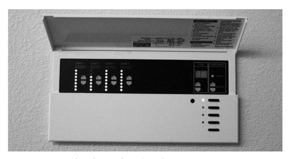
A Four Scene Four Channel Preset Dimmer (Lutron). Four Buttons Are Scenes—Four LED Ladders with Up Down Buttons Are the Four Channels, or Separately Dimmed Circuits
