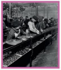
**Henry Ford** made use of the conveyor belt on the assembly line at his factory producing the Model T. Workers specialized in one task with one set of tools, which lay within easy reach.
