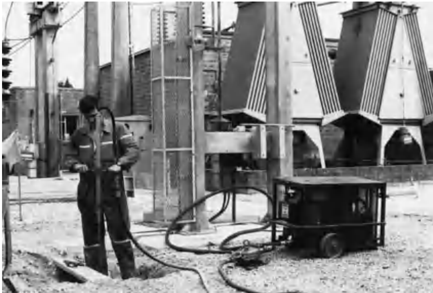
Fig. 7.10 New method showing a copper-weld earth rod driven by hydraulic 'mole' Grundomat ( T T. UK Ltd ).
