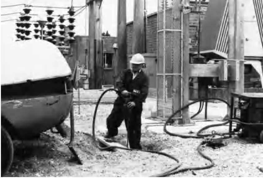
Fig. 7.11 Standard method showing copper-clad earth rod driven by a compressed air tool with compressor, as used by Stemet Earthing Co. Ltd.
