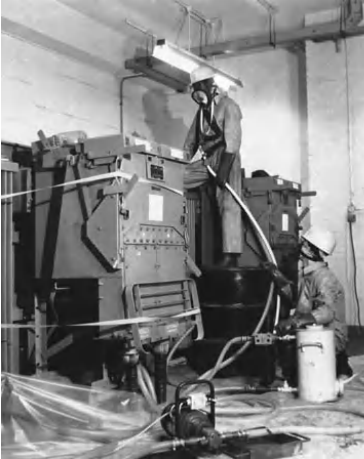
Fig. 13.3 Retrofilling of an askarel-filled unit in situ by R.F. Winder Ltd. The liquid is being replaced by silicone under carefully controlled conditions. Protective clothing is being worn by the operators.
