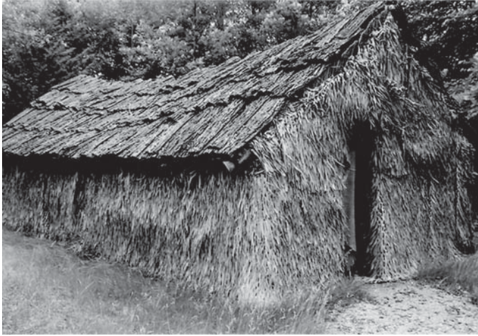
Figure 12.5. Reconstruction of a reed house located at a nature center near Spicer, Minnesota (photograph by Larry Barton).
