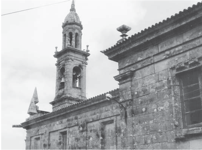
Figure 12.21. Microorganisms growing on stone; lichens and cyanobacteria growing on walls of a building in northwestern Spain (photograph by Larry Barton). See insert for color representation.
