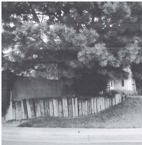
Figure 13.9. Railroad ties are used in landscaping because the creosote treatment retards microbial growth. See insert for color representation.
