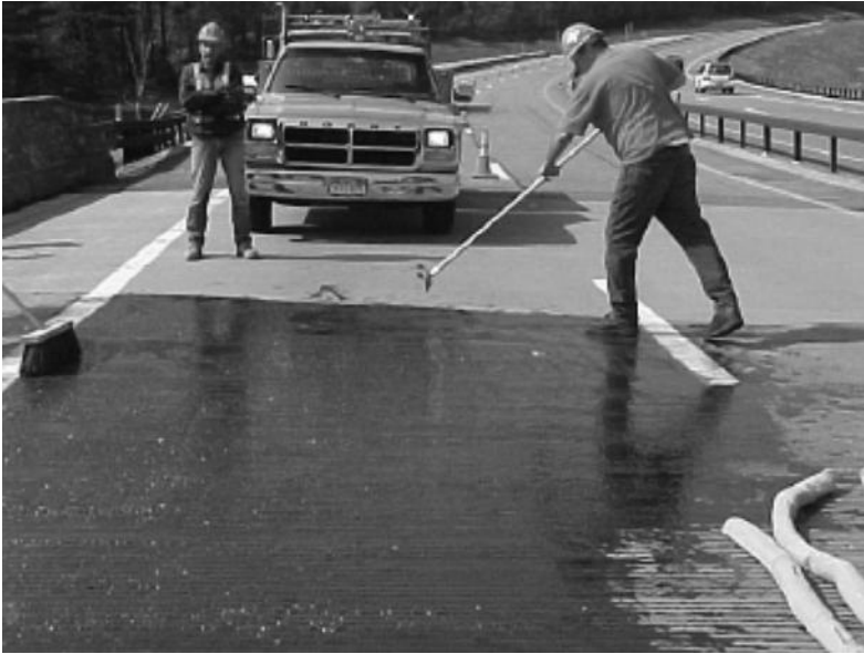
FIGURE 11.18 Concrete deck sealing. (Courtesy of the New York State Department of Transportation.)
