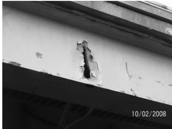
FIGURE 11.23 Damage due to vehicle collision. (Courtesy of the New York State Department of Transportation.)
