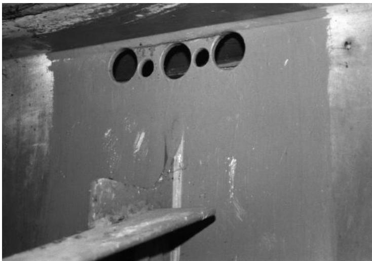
FIGURE 14.8 A repaired web gap detail with a cut-short connection plate and drilled holes.
