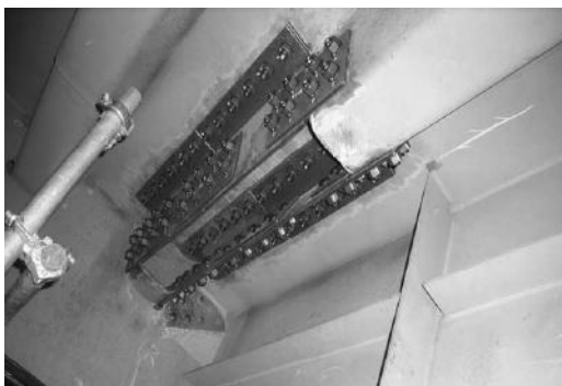
FIGURE 17.20 Partial replacement of longitudinal rib.
