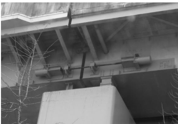
FIGURE 16.18 Seismic restrainer system.
