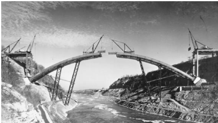
FIGURE 1.4 Lewiston-Queenston arch bridge, near Niagara Falls, New York, 1962. The longest fixed-arch span in the United States at 1000 ft. (305 m); rise is 159 ft. (48 m). Box arch-rib sections are typically about 3 \times 13 \frac{1}{2} ft. ( 0.9 \times 4.1 m) in cross-section and about 44 \frac{1}{2} ft. (13.6 m) long. Job was estimated using erection tiebacks (same as shown in Figure 1.3), but subsequent studies showed the long, sloping falsework bents to be more economical (even if less secure looking). Much permanent steelwork was used in the falsework bents. Derricks on approaches load steelwork onto material cars that travel up arch ribs. The 115-ton-capacity travelers are shown erecting the last full-length arch-rib sections, leaving only the short, closing crown sections to be erected. Canada is at left, the United States at right. (Courtesy of Bethlehem Steel Corporation.)
