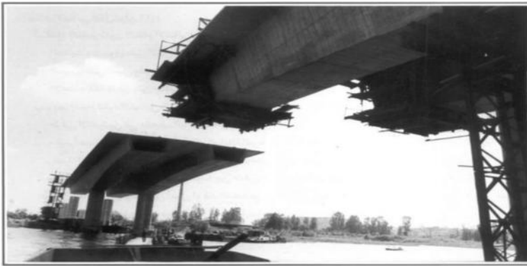
FIGURE 19.32 Casting of segment (Rod El-Farag Bridge).
