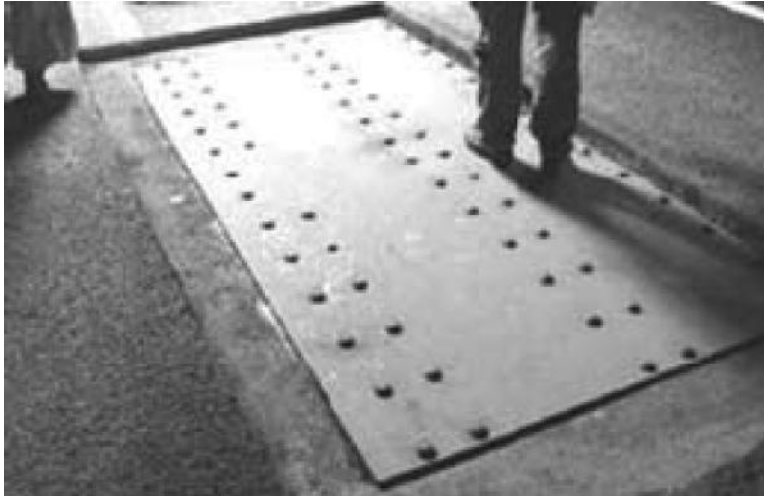
FIGURE 17.17 Plate patching for FR1-type fatigue crack.
