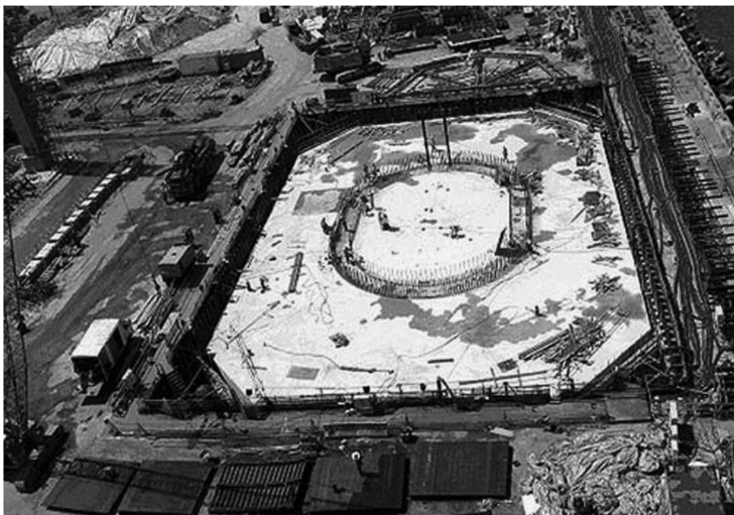
FIGURE 4.14 Tower foundation construction, Stonecutters Bridge ( http://www.zgjw.net ).
