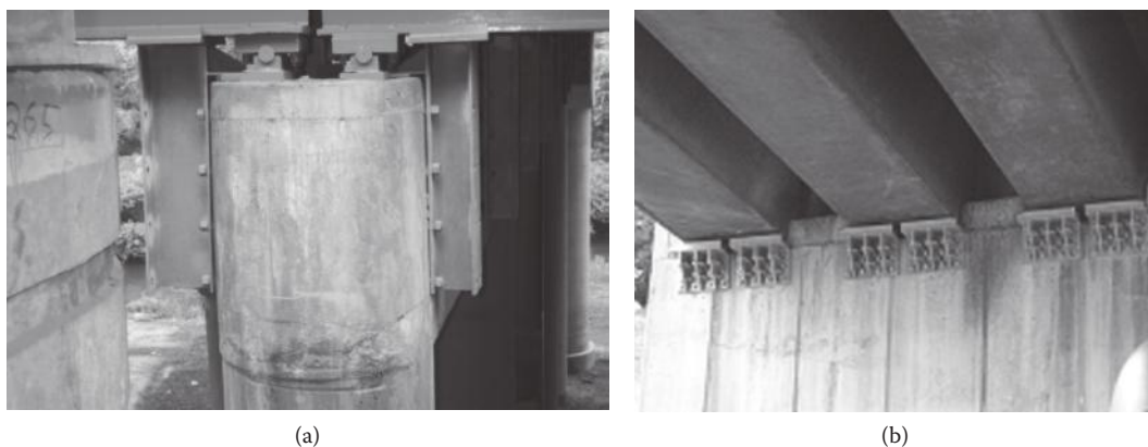
FIGURE 16.17 Seismic retrofit for insufficient seat length: (a) bumper block, (b) catcher block.
