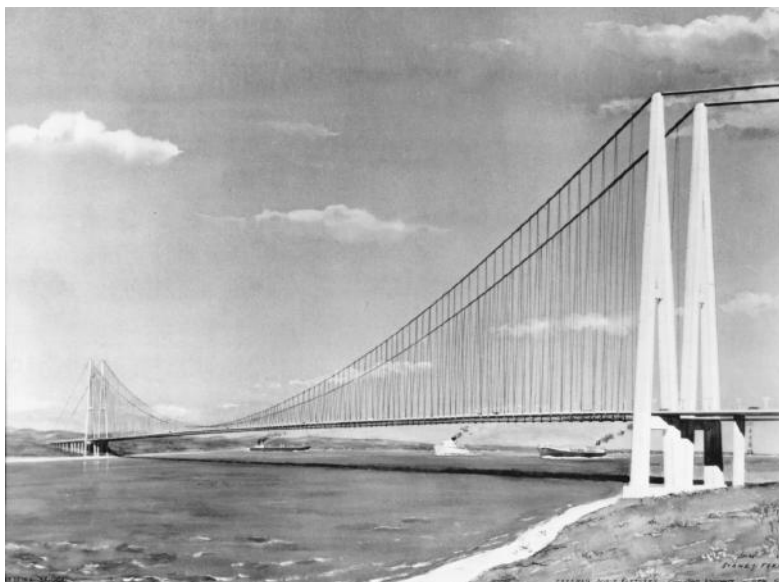
FIGURE 1.47 Artist's rendering of proposed Messina Strait suspension bridge connecting Sicily with mainland Italy. The Messina Strait crossing has been under discussion since about 1870, under investigation since about 1955, and under active design since about 1975. The first realistic proposals for a crossing were made in 1969 in response to an international competition sponsored by the Italian government. There were 158 submissions—eight American, three British, three French, one German, one Swedish, and the remaining Italian. Forty of the submissions showed a single-span or multi-span suspension bridge. The enormous bridge shown has a single span of 10,827 ft. (3300 m) and towers 1250 ft. (380 m) high. The bridge construction problems for such a span would be tremendously challenging. (Courtesy of Stretto di Messina, S.p.A.)
