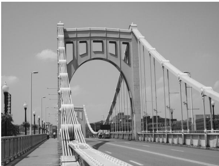
FIGURE 13.7 Fracture critical bridge superstructure.
