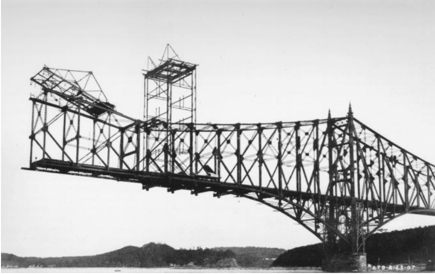
FIGURE 1.11 First Quebec railway cantilever bridge, August 23, 1907. Cantilever erection of south main span, 6 days before collapse. The tower traveler erected the anchor span (on falsework) and then the cantilever arm; then erected the top-chord traveler, which is shown erecting suspended span at end of cantilever arm. The main span of 1800 ft. (549 m) was the world's longest of any type. The sidespan bottom chords second from pier failed in compression because latticing connecting chord corner angles was deficient under secondary bending conditions.
