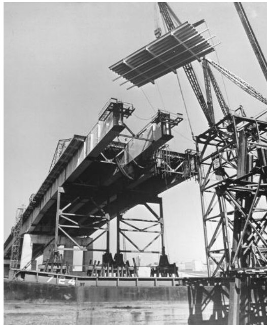
FIGURE 1.36 Erecting orthotropic-plate decking panel, Poplar Street Bridge, St. Louis, Mo., 1967. A five-span, 2165 ft. (660 m) continuous box-girder bridge, main span 600 ft. (183 m). Projecting box ribs are 5\frac{1}{2} \times 17 ft. ( 1.7 \times 5.2 m) in cross-section, and decking section is 27 \times 50 ft. ( 8.2 \times 15.2 m). Decking sections were field welded, while all other connections were field bolted. Box girders are cantilevered to falsework bents using overhead “positioning travelers” (triangular structure just visible above deck at left) for intermediate support. (Courtesy of Bethlehem Steel Corporation.)
