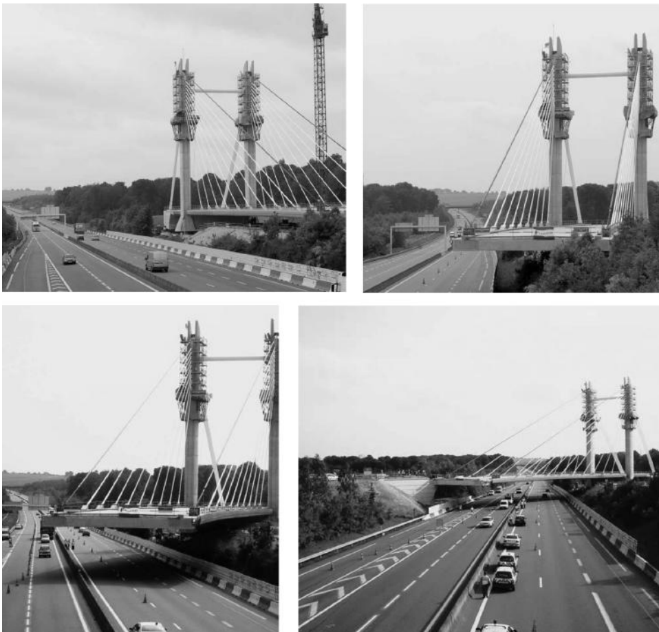
FIGURE 19.54 Example of bridge rotation (Freyssinet).
