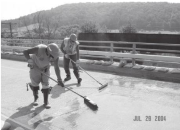
Spreading the polymer material
