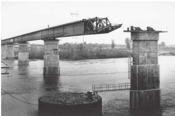
FIGURE 1.41 Erection of Kansas City Southern Railway box-girder bridge, near Redland, Okla., by “launching,” 1970. This nine-span continuous box-girder bridge is 2110 ft. (643 m) long, with a main span of 330 ft. (101 m). Box cross section is 11 × 14.9 ft. (3.35 × 4.54 m). Girders were launched in two “trains,” one from north end and one from south end. A “launching nose” was used to carry leading end of each girder train up onto skidway supports as train was pushed out onto successive piers. Closure was accomplished at center of main span. (a) Leading end of north girder train moves across 250 ft. (76 m) span 4, approaching pier 5. Main span, 330 ft. (101 mm), is to right of pier 5.
