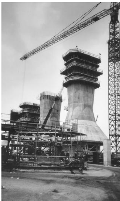
FIGURE 6.26 Prefabricated pier shaft and icebreaker for the Prince Edward Island Bridge.
