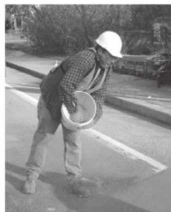
Placing aggregate
