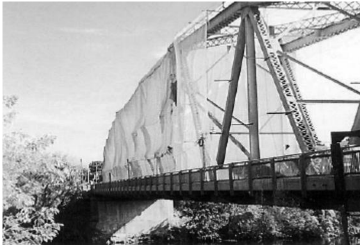
FIGURE 11.20 Bridge painting. (Courtesy of the New York State Department of Transportation.)
