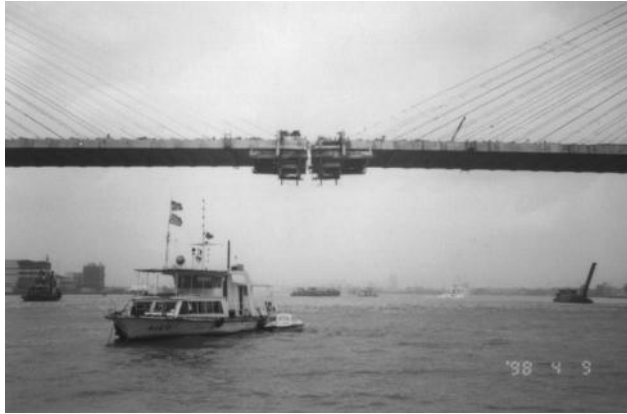
FIGURE 5.15 Two cantilever ends are meeting very well.
