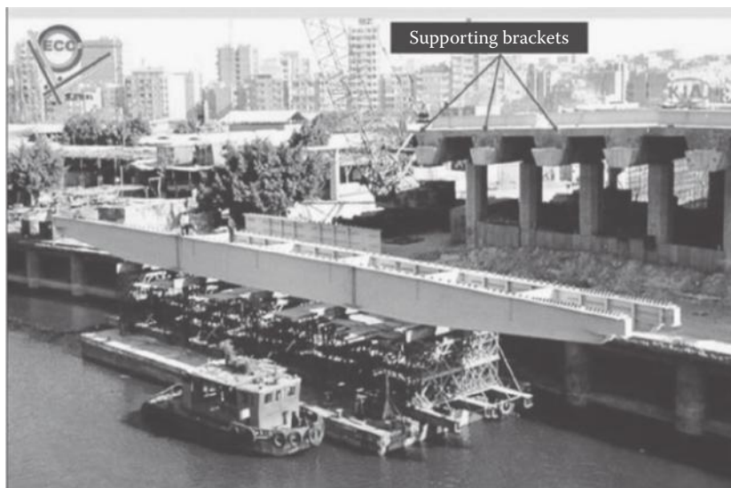
FIGURE 19.46 Steel beams to be supported by the brackets (El-Moneeb Bridge).
