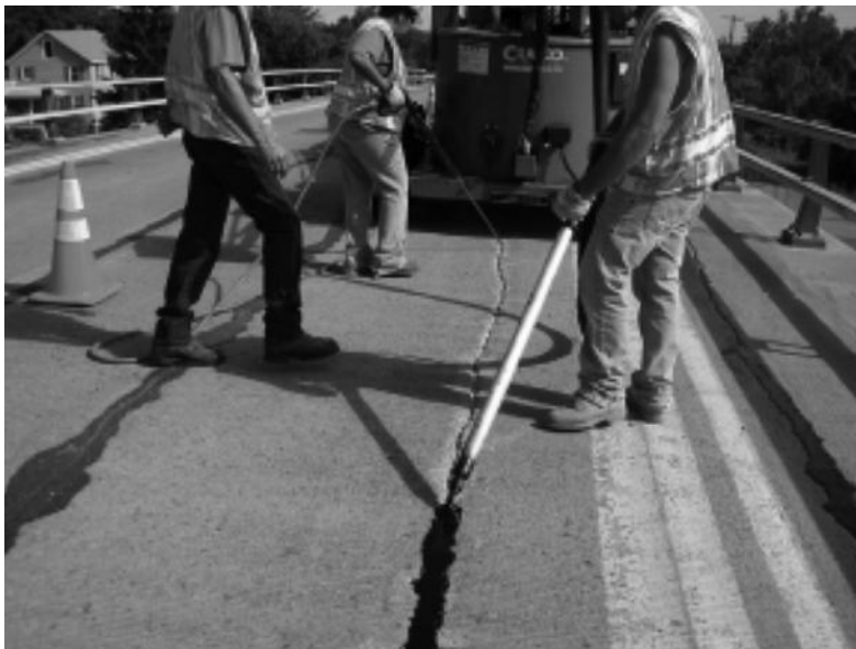
FIGURE 11.17 Crack sealing. (Courtesy of the New York State Department of Transportation.)
