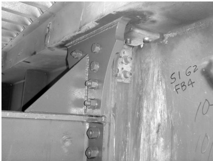
FIGURE 14.11 Repair of distortion-induced fatigue using field welding.
