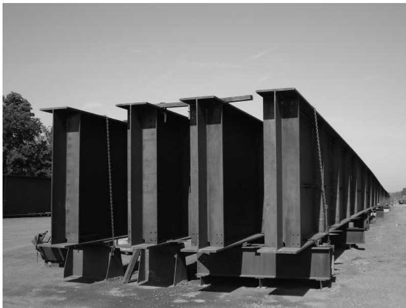
FIGURE 2.7 Girders in line assembly. Such assembly may be accomplished with the girders vertical, as shown, or horizontal, in the “lay down” position.
