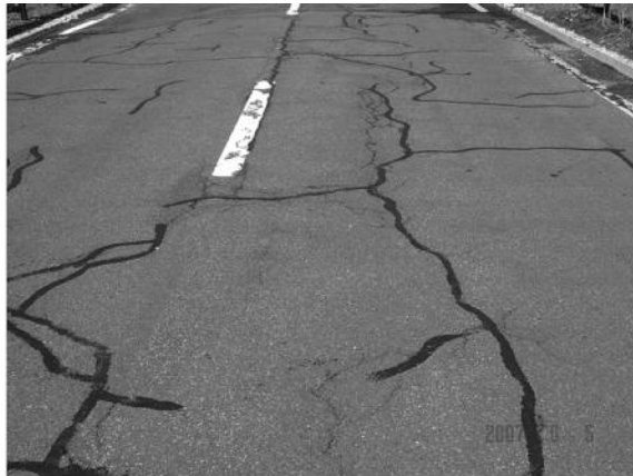
FIGURE 11.23 Damage due to vehicle collision. (Courtesy of the New York State Department of Transportation.)
