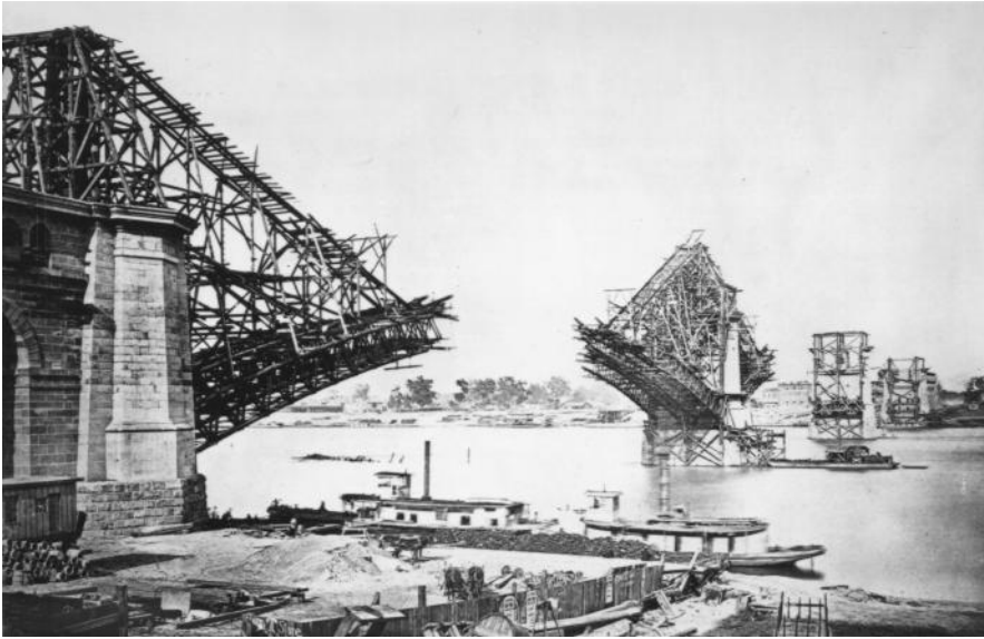
FIGURE 1.15 Eads Bridge across the Mississippi River, St. Louis, Mo., 1873. The first important metal arch bridge in the U.S., it is supported by four planes of hingeless trussed arches having chrome-steel tubular chords. Spans are 502-520-502 ft. (153-158-153 m). During erection, arch trusses were tied back by cables passing over temporary towers built on the piers. Arch ribs were packed in ice to effect closure.
