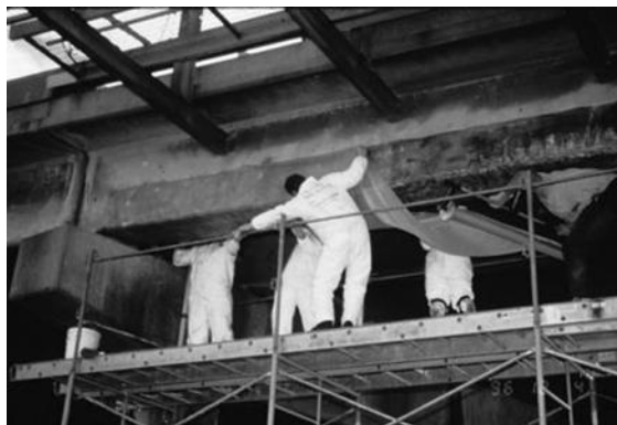
FIGURE 16.26 Glass fiber-reinforced polymer fabric to strengthen deteriorated reinforced concrete T-beam. (Courtesy of FHWA.)
