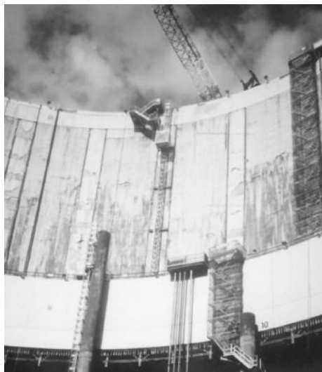
FIGURE 6.11 Concrete ring wall cofferdam constructed by slurry trench methods.
