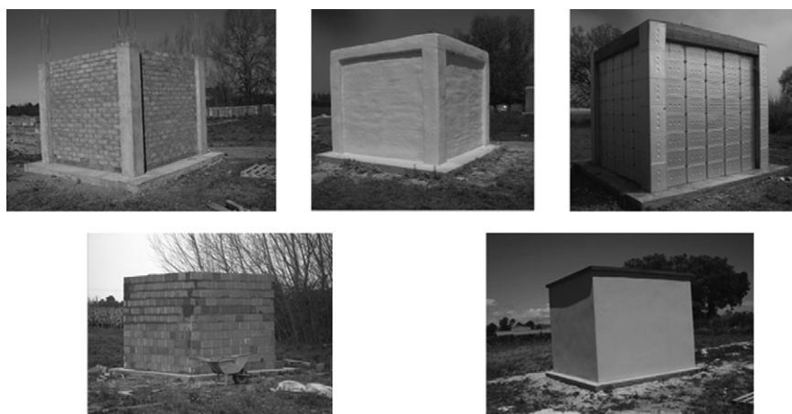
13.2 Brick cubicles: construction process.
