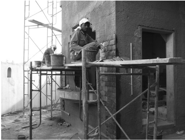
20.3 Stone cladding layers.
