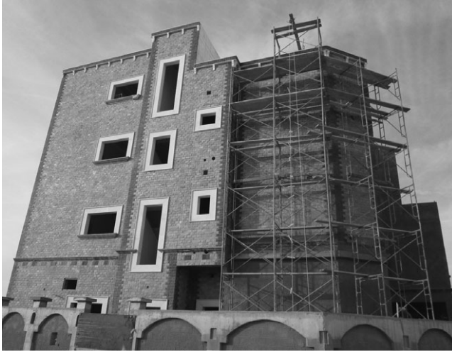
20.4 A typical Bahraini residential building.
