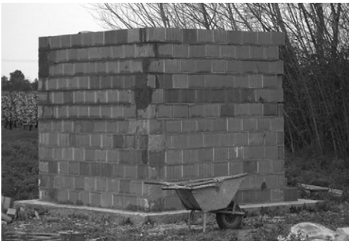
13.6 Alveolar brick cubicles: construction phase.
