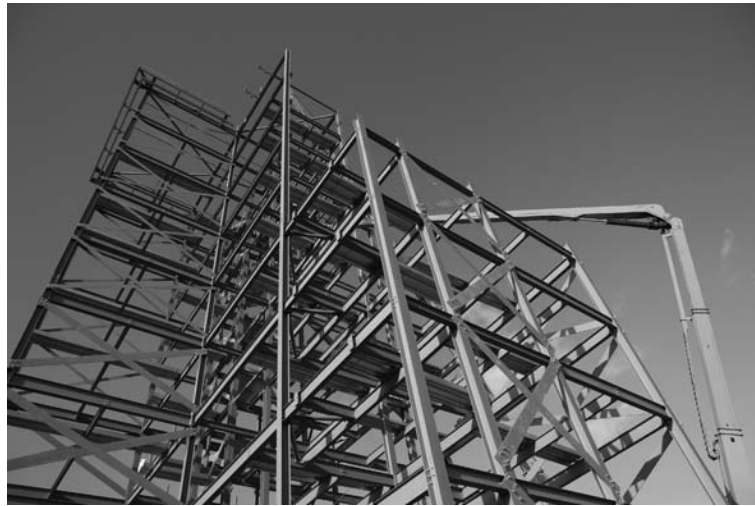
Fig. 1.4 Skeleton of a Structural Steel Frame Building
