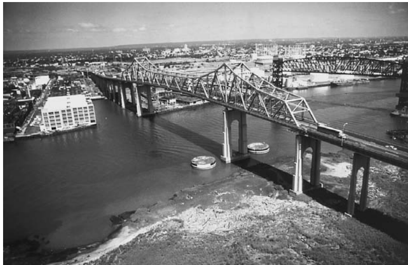
Goethals Bridge, a Cantilever Truss Bridge between Staten Island, NY, and Elizabeth, NJ.
