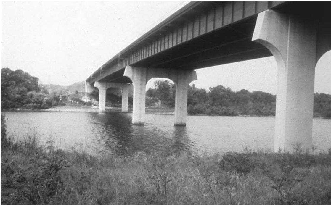
A Continuous Beam Bridge
