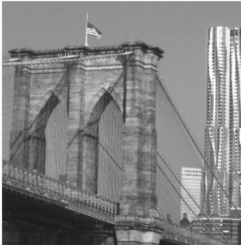
Beekman Tower and Brooklyn Bridge, New York
