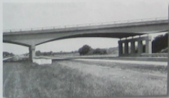
A continuous, reinforced-concrete highway bridge.
