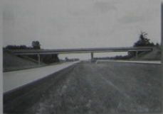
These bridge girders are statically indeterminate since they are continuous over their piers.
