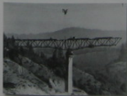
A truss bridge being constructed over Lake Shasta in northern California.
