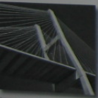
Cable-stayed bridge in Savannah, Georgia.
