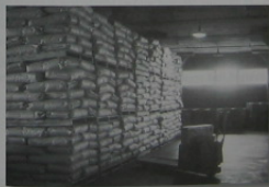
The design of the floor system of this warehouse building must account for critical locations of storage materials on the floor. Influence lines must be used for this purpose. (Photo courtesy of Portland Cement Association.)
