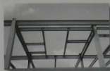
The portion of a slab supported between the floor beams and girders of this structural system will transmit its load either by one- or two-way action depending upon its L_1 and L_2 dimensions.
