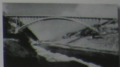
An example of a two-ribbed, open-spandrel fixed-arch bridge having a main span of 1000 ft (304 m). (Courtesy of Bethlehem Steel Corporation.)
