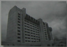
The shear walls on the sides of this building are used to strengthen the structure when it is subjected to large wind loadings applied to the front or back of the building.
