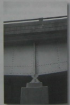
Typical pin used to support the steel girder of a railroad bridge.
