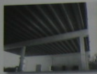
The many concentrated loadings acting on this reinforced concrete beam create a variation of the internal loading in the beam. For this reason, the shear and moment diagrams must be drawn in order to properly design the beam.
