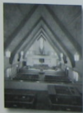
Timber frames having a variable moment of inertia are often used in the construction of modern churches.
