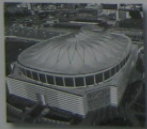
The roof of the "Georgia Dome" in Atlanta, Georgia can be considered as a thin membrane.
