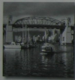
Parker trusses are used to form this bridge.
