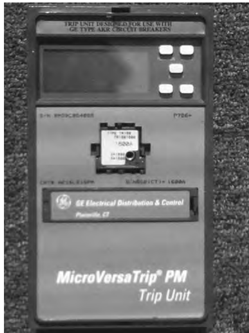
FIGURE 8.2 Micro-VersaTrip Plus, static-trip device.
