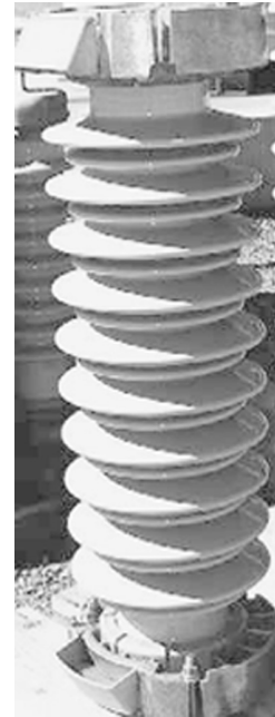
FIGURE 10.8 Post insulators.
