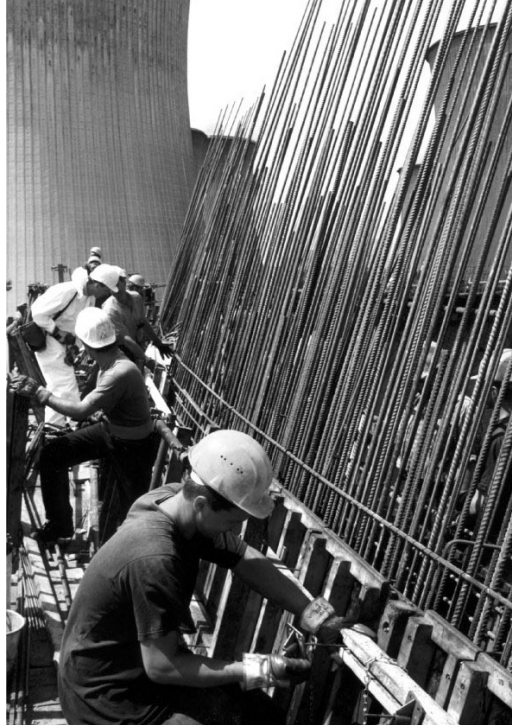
FIGURE 27.7 Formwork and steel reinforcement of shell wall.
