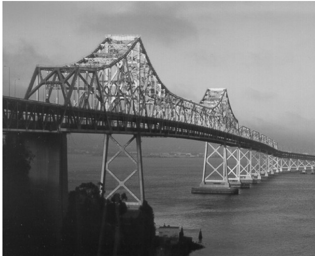
FIGURE 25.6 San Francisco-Oakland Bay Bridge — east span.
