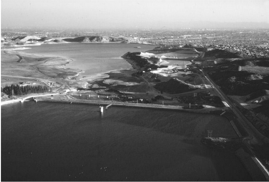
FIGURE 18.23 Aerial view of Lower San Fernando Dam and San Fernando Valley. (Photograph courtesy of Steinbrugge Collection, Earthquake Engineering Research Center, University of California, Berkeley.)
