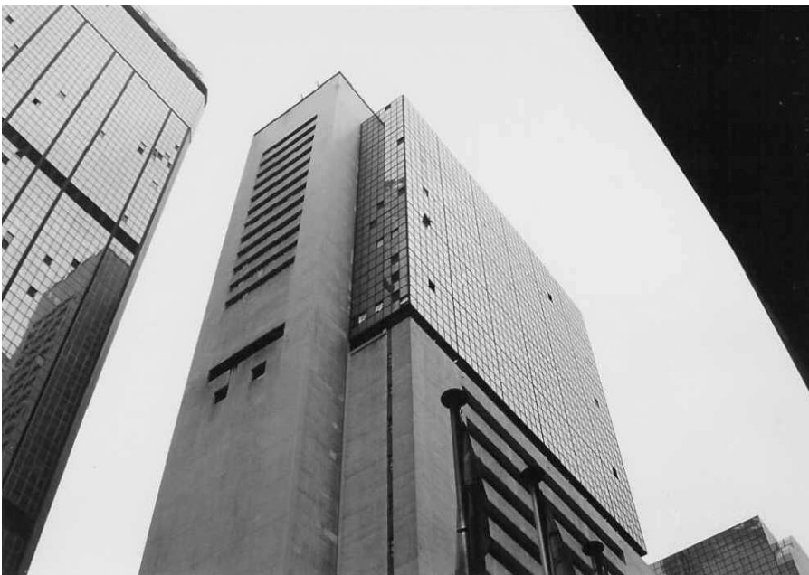
FIGURE 29.3 Damage of buildings after a typhoon attack.
