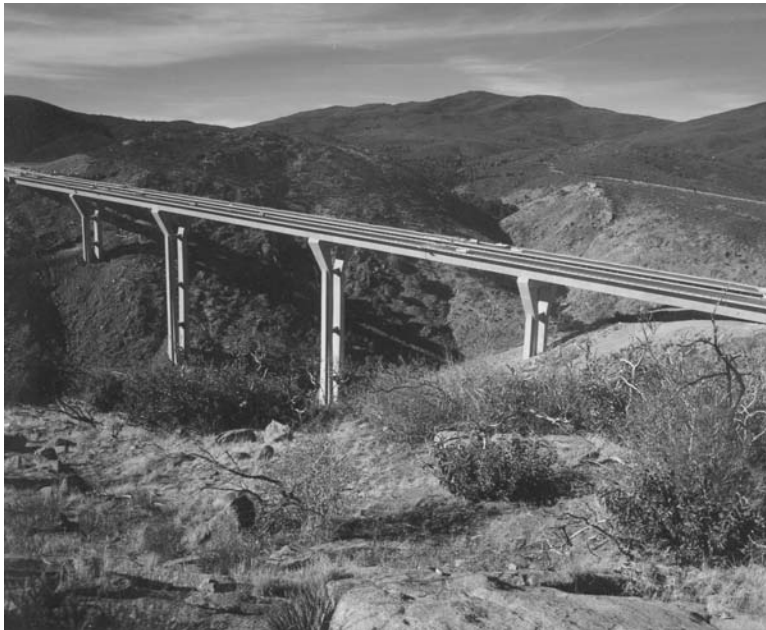
FIGURE 25.38 Pine Valley Bridge — construction completed, California.
