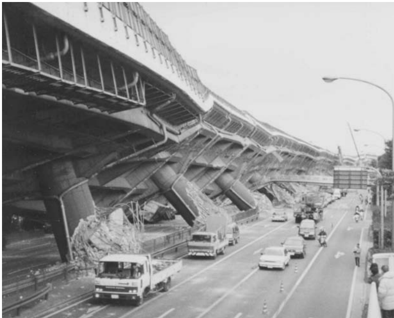
FIGURE 20.3 Collapse of Hanshin Expressway in the 1995 Hyogo-Ken Nanbu Earthquake in Japan (courtesy of Mark Yashinsky).
