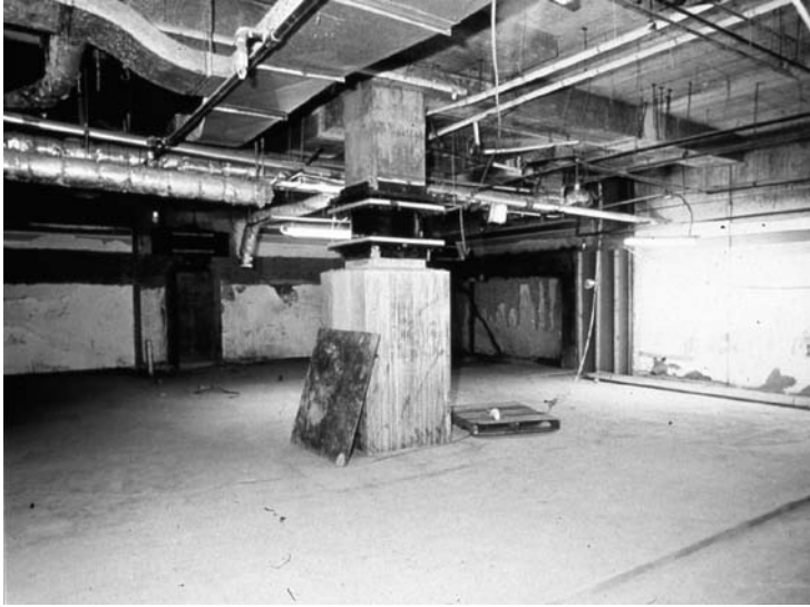
FIGURE 18.85 The concrete columns were cut at midheight and lead-rubber isolation devices were installed. (Photo courtesy of Dynamic Isolation Systems Inc.)
