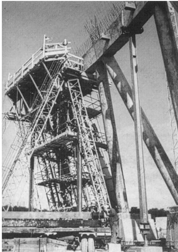
FIGURE 27.5 Fabrication of supporting columns.
