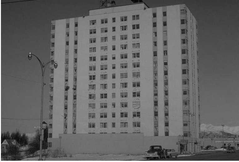
FIGURE 18.48 West elevation of the Mt. McKinley Apartment building after the 1964 Great Alaska Earthquake. (Photograph by Karl Steinbrugge, Earthquake Engineering Research Center, University of California, Berkeley.)
