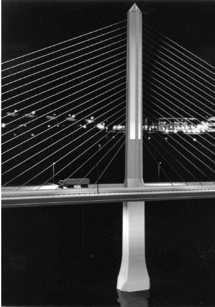
PHOTO 8.1 A rendering of the new Maumee River Bridge, Toledo, Ohio. This cable-stayed bridge spans the Maumee River in downtown Toledo as a monument icon for the city. The design includes single pylon, single plane of stays, and a main span with a horizontal clearance of 612 ft in both directions. The main pylon is clad on four of its eight sides with a glass curtain wall system, symbolizing the glass industry and heritage of Toledo. This glass prismatic system and stainless steel clad cables create a sleek and industrial look during the day. At night, the glass becomes very dynamic with the use of LED arrays back-lighting the window wall. Owner: Ohio Department of Transportation (courtesy of the Designer, Figg Engineering Group, Linda Figg, President, Tallahassee, Florida).
