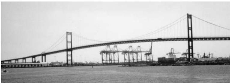
FIGURE 18.87 The Vincent Thomas Bridge is a three-span suspension structure built over the port of Los Angeles.
