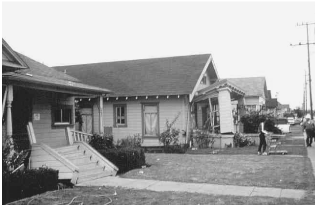
FIGURE 10.5 Houses damaged due to cripple wall failure, 1983 Coalinga Earthquake (courtesy of EQE International).
