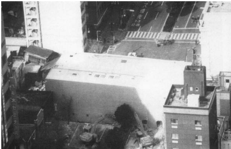
FIGURE 18.42 Eventual collapse of nine-story SRC building after the Kobe Earthquake. (Photo courtesy of NIST; NIST, The January 17, 1995 Hyogoken-Nanbu (Kobe) Earthquake, U.S. NIST, Gaithersburg, MD, 1996.)
