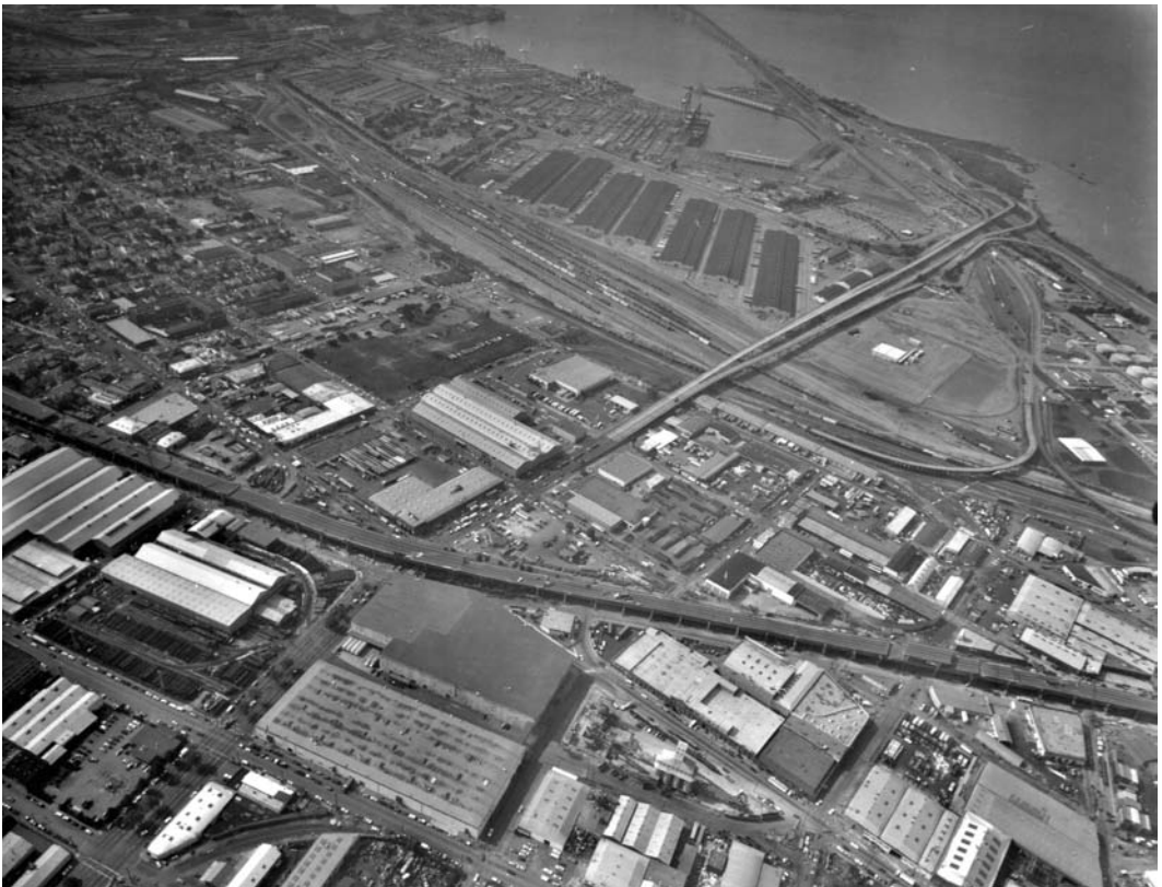
FIGURE 18.29 Aerial view of Cypress Viaduct showing collapse where the structure crossed over Bay mud.
