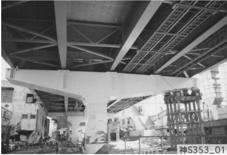
FIGURE 18.68 Collapsed building leaning against the Kobe Route 3 Expressway. (Photo courtesy of Hanshin Expressway Public Corporation.)
