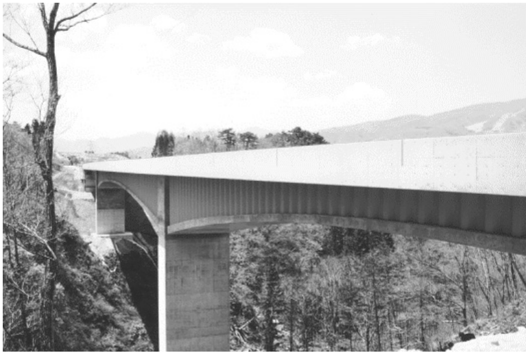
FIGURE 25.39 Prestressed concrete bridge with corrugated steel web (Hondani Birdge, Japan, from P.S. Mitsubishi Construction Co. Ltd., with permission).
