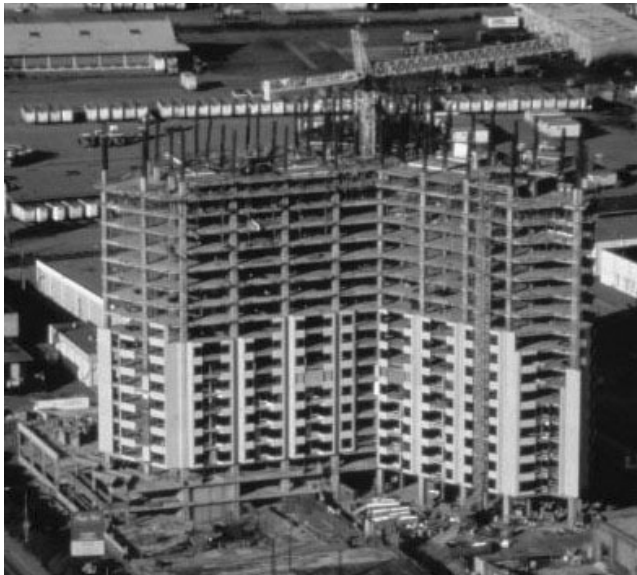
PHOTO 7.1 A 30-story reinforced concrete building under construction. The Pacific Park Plaza is one of the largest reinforced concrete structures in the San Francisco Bay area. It survived the October 17, 1989, Loma Prieta earthquake without damage. Instrumentation in the building recorded peak horizontal accelerations of 0.22g at the base and 0.39g at the top of the building (courtesy of Mr. James Tai, T.Y. International, San Francisco).
