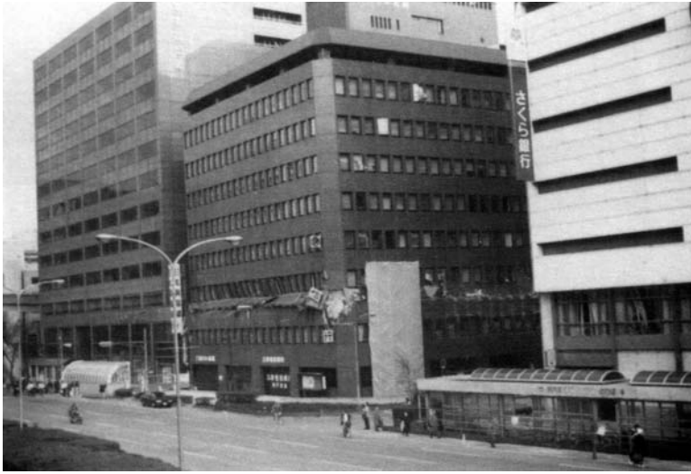
FIGURE 18.39 Ten-story SRC building with third floor collapse during the Kobe Earthquake. (Photo courtesy of NIST; NIST, The January 17, 1995 Hyogoken (Kobe) Earthquake, U.S. NIST, Gaithersburg, MD, 1969.)
