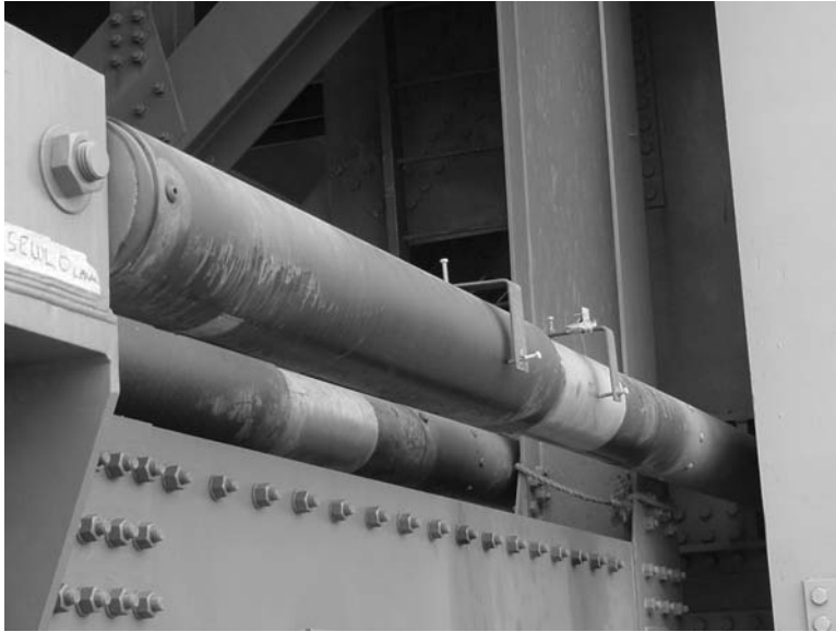
FIGURE 18.88 The Vincent Thomas Bridge retrofit provided gaps between the decks and the towers and also fluid viscous dampers to dissipate energy. (Photo courtesy of Enidine Inc.)
