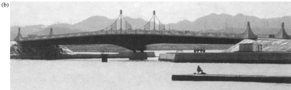
FIGURE 25.57 Pedestrian railing (JASBC 1985): (a) railing images waves and (b) Kanazawa Kakkei Oh-Hashi, Kanagawa, Japan (1982).
