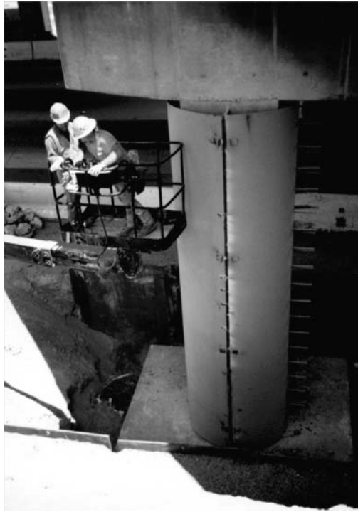
FIGURE 18.89 Steel shell being wrapped around a concrete bridge column to increase its ductility and shear strength.
