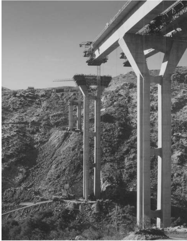
FIGURE 25.37 Pine Valley Bridge — construction stage, California.
