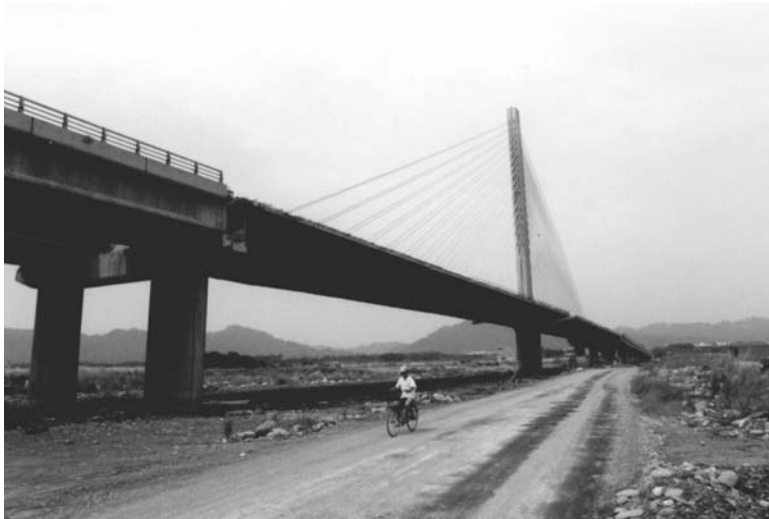
FIGURE 18.44 The Ji Lu cable-stayed bridge after the 1999 Ji Ji, Taiwan, earthquake.
