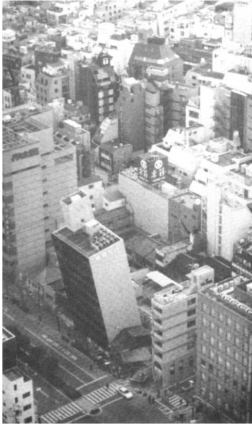
FIGURE 18.41 Nine-story SRC building immediately after the 1995 Kobe Earthquake. (Photo courtesy of NIST; NIST, The January 17, 1995 Hyogoken-Nanbu (Kobe) Earthquake, U.S. NIST, Gaithersburg, MD, 1996.)
