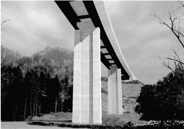
FIGURE 25.23 Widely spaced girder bridge (Chidorinosawagawa Bridge, Japan, from Kawasaki Heavy Ind., Ltd., with permission).
