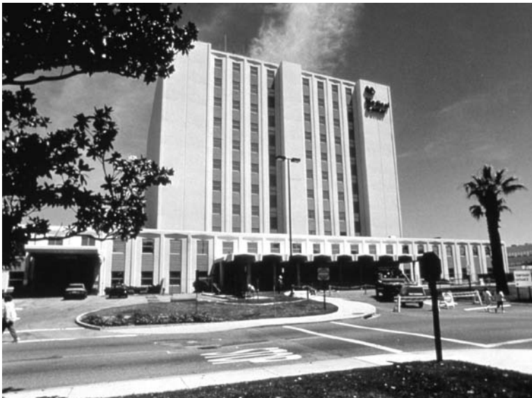
FIGURE 18.84 The existing Long Beach VA Hospital was seismically retrofit with lead-rubber bearings. (Photo courtesy of Dynamic Isolation Systems, Inc.)
