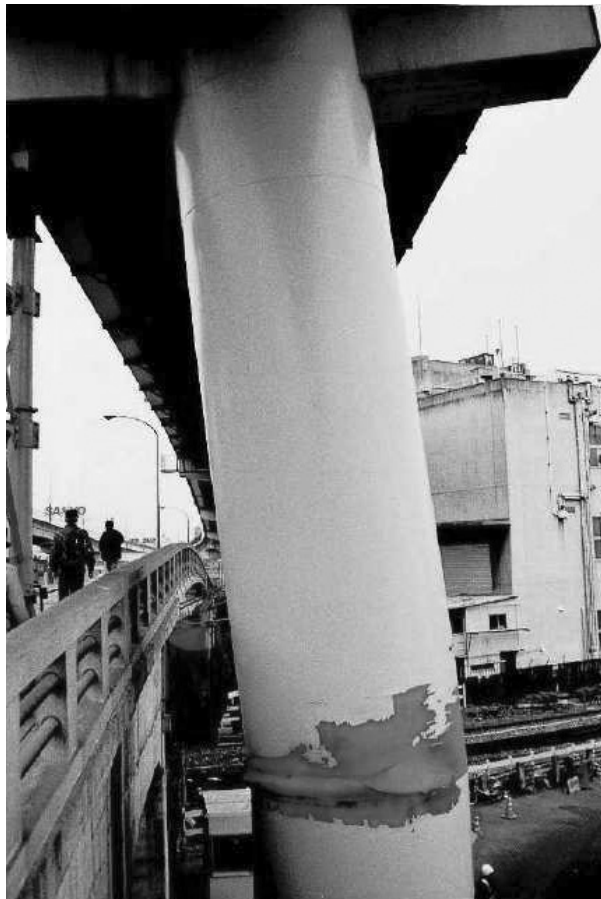
FIGURE 18.54 Pier 585 on Kobe Route 3 during the 1995 Kobe Earthquake. (Photo courtesy of Hanshin Expressway Public Corporation.)
