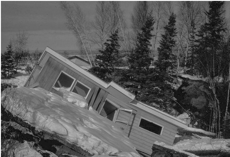
FIGURE 18.18 About 75 homes were damaged as a result of the Turnagain Heights Slide. (Photograph courtesy of Steinbrugge Collection, Earthquake Engineering Research Center, University of California, Berkeley.)
