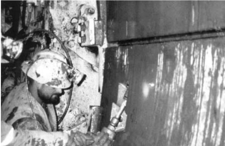
FIGURE 28.8 Installation of one-pass liner (© Bernie Martin, with permission).
