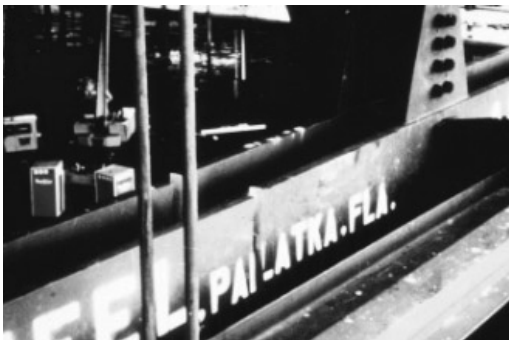
FIGURE 34.18 Jumbo section used as tension chord in a roof truss and fracture in web originating from weld access holes at welded splice.
