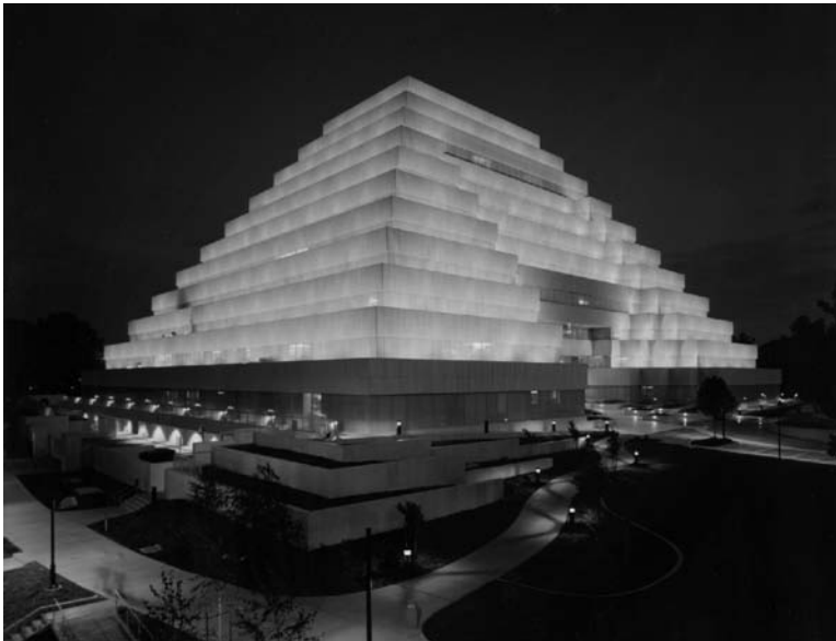
FIGURE 18.81 The uniquely shaped "Money Store" was designed with fluid viscous dampers to improve its seismic behavior. (Photo courtesy of Marr-Shaffer & Miyamoto, Structural Engineers.)
