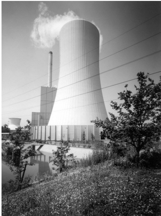
FIGURE 27.55 Coated cooling tower shell at Herne Power Station, Germany.
