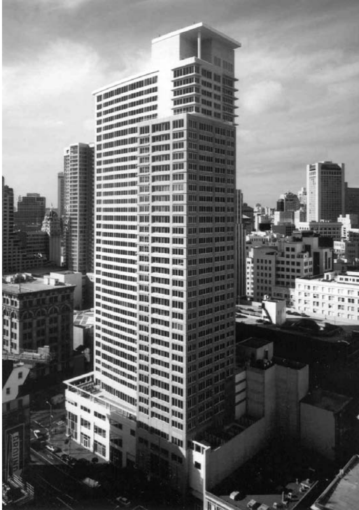
PHOTO 8.4 Paramount Apartments, San Francisco, CA: completed in 2002, it is the first hybrid precast prestressed concrete moment-resistant 39 floor high-rise frame building in a high seismicity zone. Based on tests of large-scale prototype of the moment-resisting connections, it was determined that the performance of the system was superior to cast-in-place concrete, both in cracking behavior and ductility. Hence, as a system, this new development succeeds in enhancing the performance of high-rise buildings and bridges in high seismicity earthquake zones. Since completion of this structure, several other buildings in California have been completed using the same principles (courtesy Charles Pankow Ltd, Design/Build contractors. Structural Engineers: Robert Englekirk Inc.).
