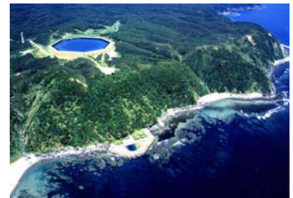
Figure 26.11. Okinawa pumped-storage power plant, whose lower reservoir is the ocean. Energy stored: 0.2 GWh. Photo by courtesy of J-Power. www.ieahydro.org .
