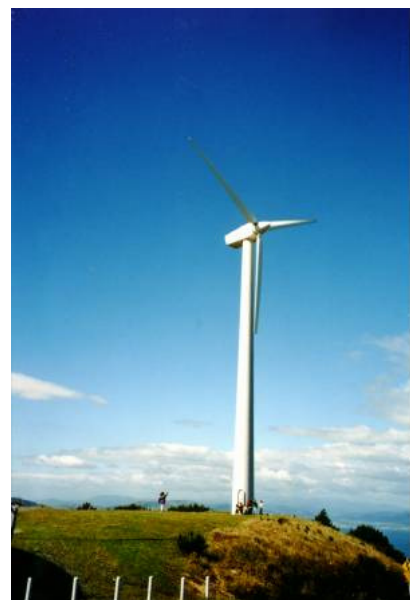
Figure B.3. The Brooklyn windmill above Wellington, New Zealand, with people providing a scale at the base. On a breezy day, this windmill was producing 60 kW, (1400 kWh per day). Photo by Philip Banks.
