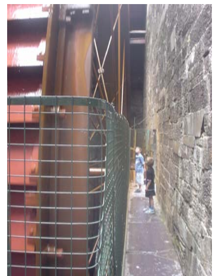
Figure 8.4. A 60 kW waterwheel.
