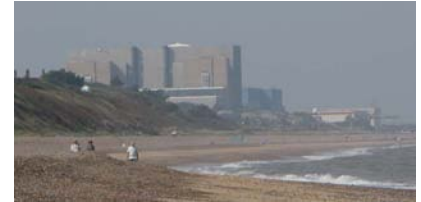
Figure 24.9. Sizewell's power stations. Sizewell A, in the foreground, had a capacity of 420 MW, and was shut down at the end of 2006. Sizewell B, behind, has a capacity of 1.2 GW. Photo by William Connolley.
