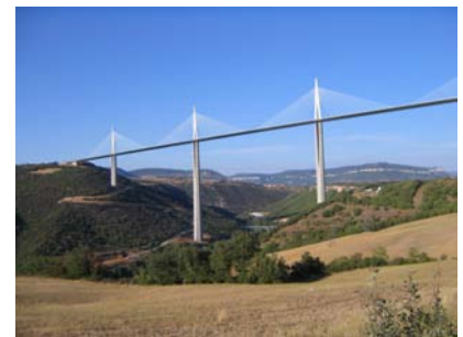
Figure H.7. Millau Viaduct in France, the highest bridge in the world. Steel and concrete, 2.5 km long and 353 m high.
