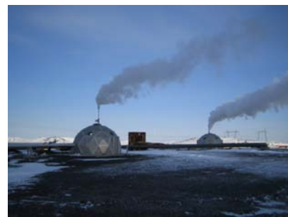
Figure 25.11. More geothermal power in Iceland. Photo by Rosie Ward.
