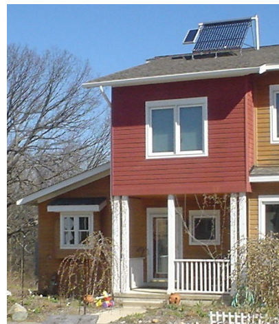
Figure 30.2. A solar water heater providing hot water for a family in Michigan. The system's pump is powered by the small photovoltaic panel on the left.
