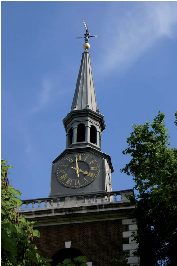
Fig. 11.2 GRP replacement spire – Church of St James, London. Photograph: Courtesy of Smith of Derby Ltd
