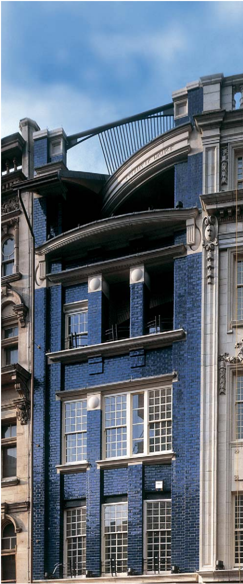
Fig. 1.9 Glazed bricks – Atlantic House, London. Architects: Proun Architects. Photograph: Courtesy of Ibstock Brick Ltd
