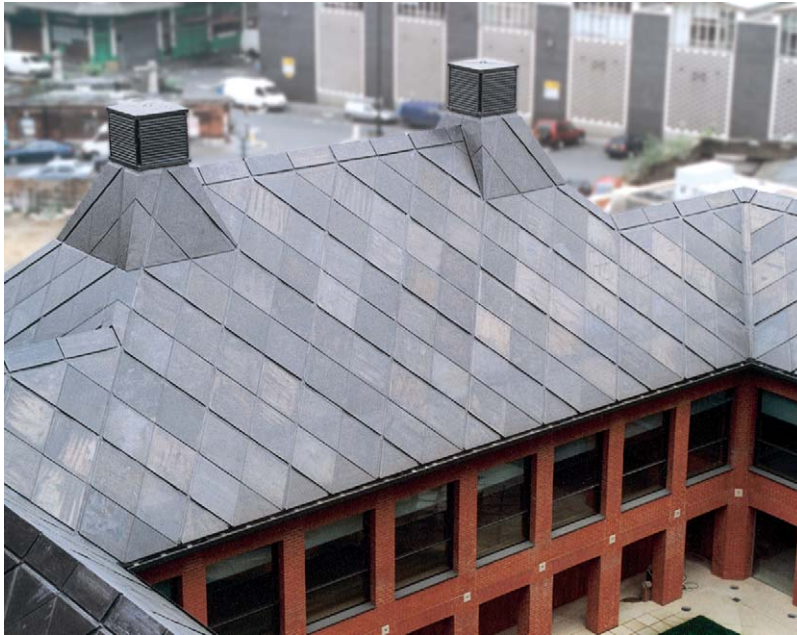
Fig. 5.27 Lead tile roofing – Haberdashers' Hall, London. Architects: Hopkins Architects. Photograph: Courtesy of Lead Contractors Association
