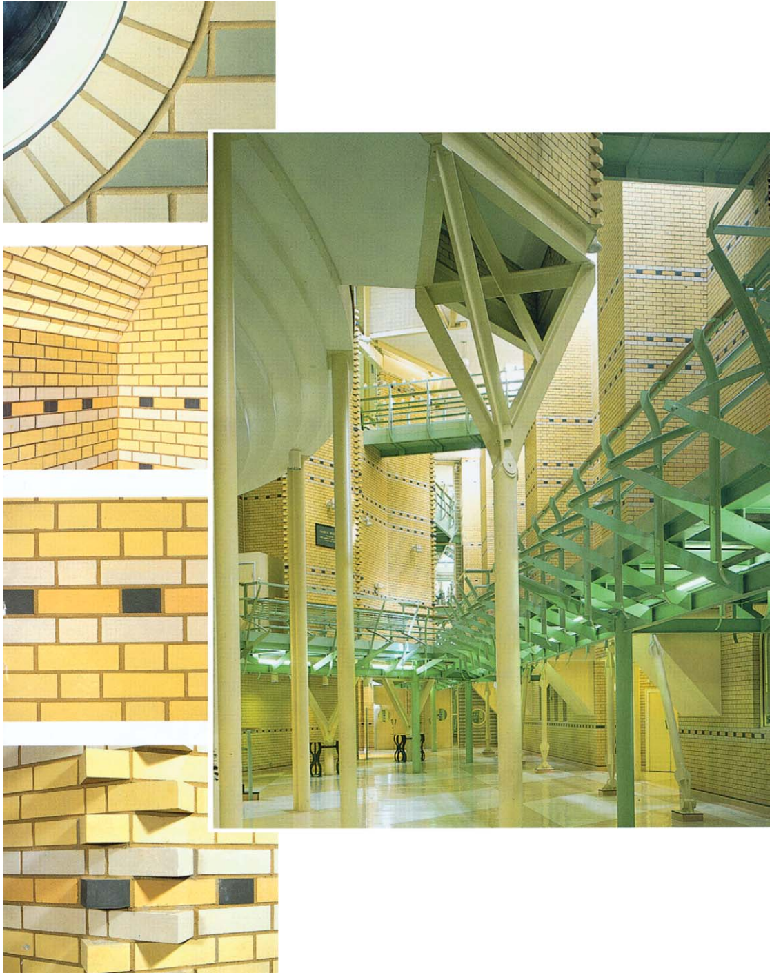
Fig. 1.21 Polychromatic calcium silicate brickwork – Queens Building, De Montfort University, Leicester. Architects: Short Ford & Associates. Photographs: Lens-based media, De Montfort University
