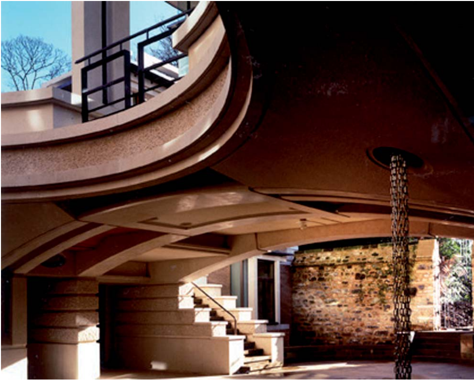
Fig. 3.16 High-quality visual concrete – St John's College, Oxford. Architects: MacCormac Jamieson Prichard. Photograph: Courtesy of Peter Cook
