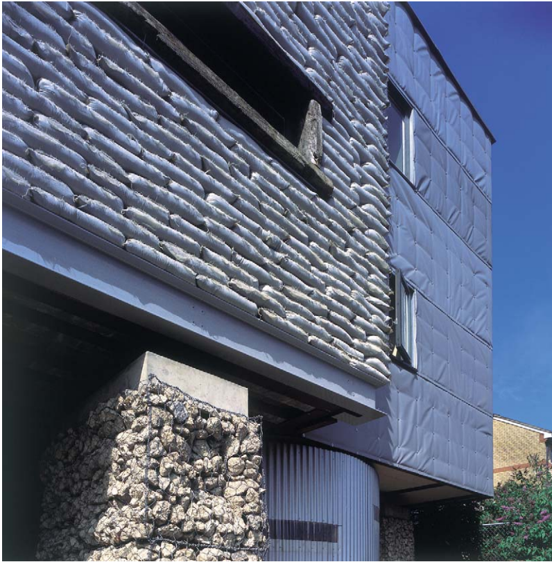
Fig. 15.6 Sandbags in construction. Architects and Photographer: Sarah Wigglesworth Architects
