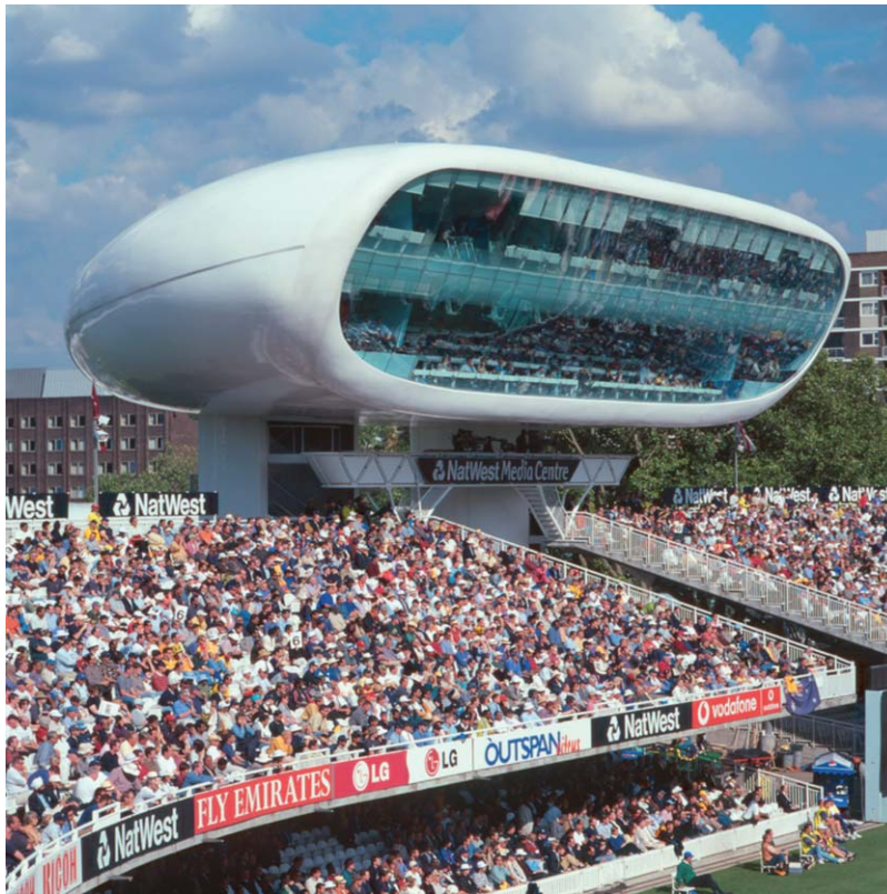
Fig. 5.19 Aluminium semi-monocoque construction – Lord's Media Centre, London. Architects: Future Systems. Photograph: Courtesy of Richard Davies
