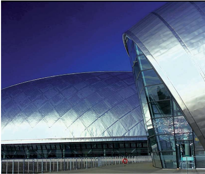
Fig. 5.30 Titanium cladding – The Glasgow Science Centre. Architects: BDP – Building Design Partnership. Photograph: Courtesy of Don Clements
