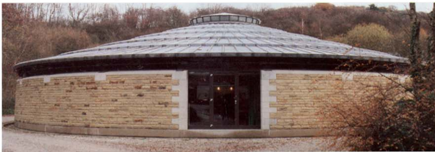
Fig. 9.10 Load-bearing stone masonry – David Mellor Cutlery Factory, Hathersage, Derbyshire. Architects: Hopkins Architects. Photographs: Arthur Lyons
