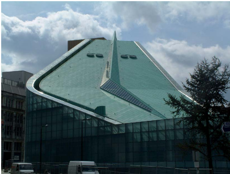
Fig. 5.21 Copper roof construction – Urbis Centre, Manchester. Architects: Ian Simpson Architects. Photograph: Courtesy of Chris Hodson
