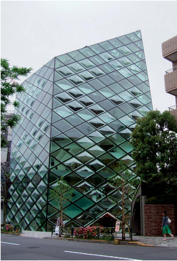
Fig. 7.12 Curved rhomboidal glass panes – Prada Store, Tokyo. Architects: Herzog and de Meuron. Photograph: Courtesy of Sam Glynn
