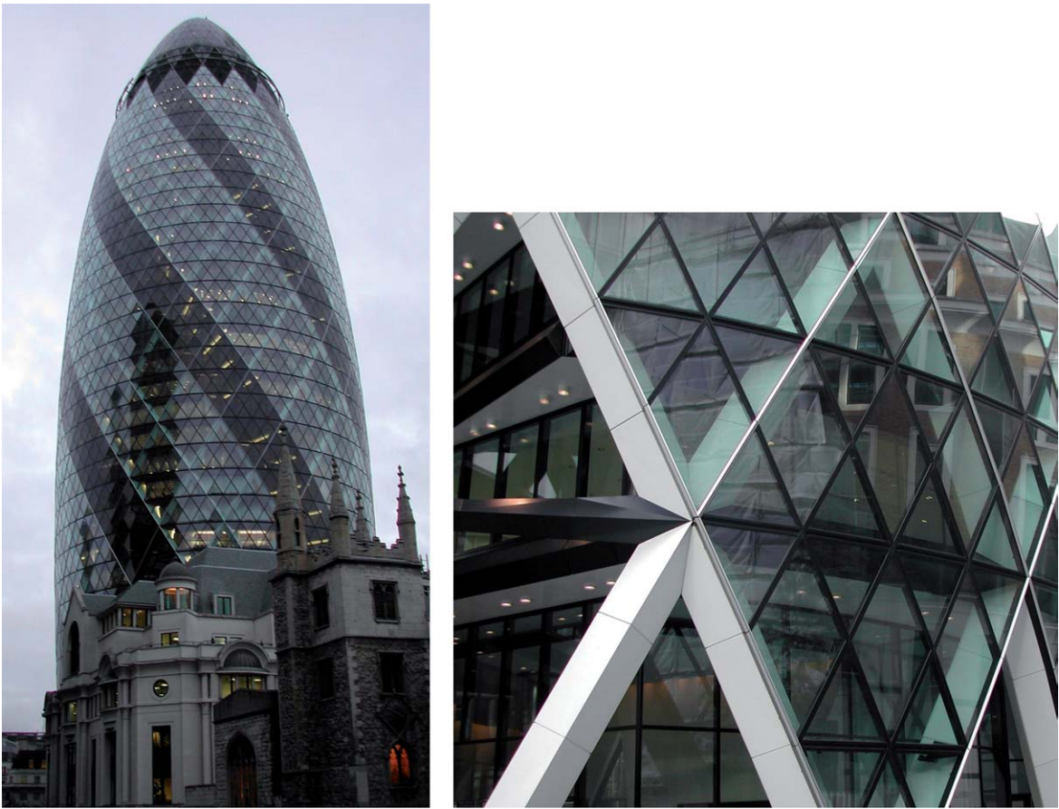
Fig. 7.16 Glazing and detail – Swiss Re Building, London. Architects: Foster and Partners. Photographs: Arthur Lyons
