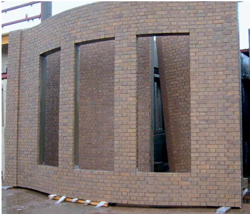
Fig. 1.17 Preassembled brickwork. Photograph: Courtesy of Trent Concrete Ltd
