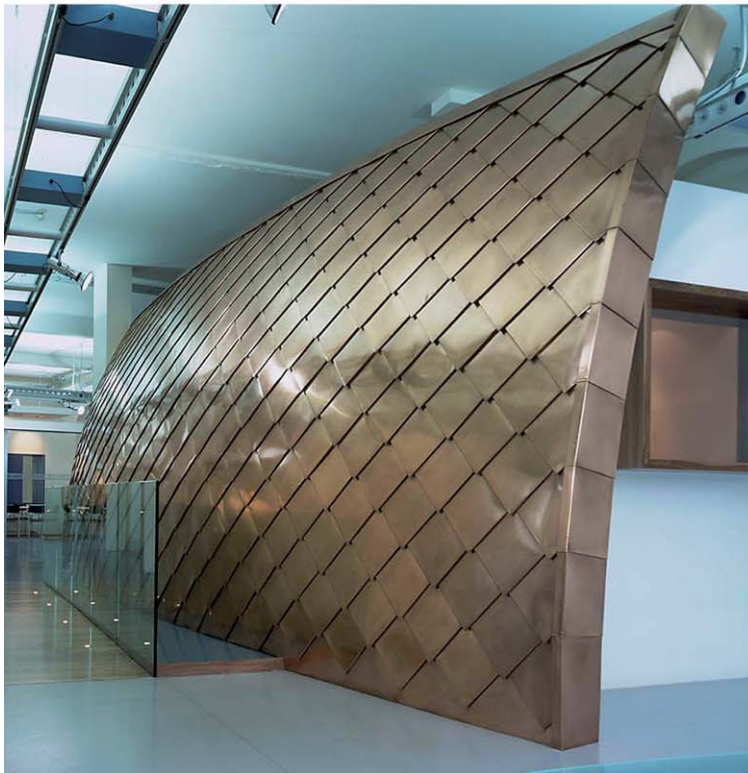
Fig. 5.23 Traditional copper roofing and copper shingles. Photograph: Courtesy of Copper Development Association
