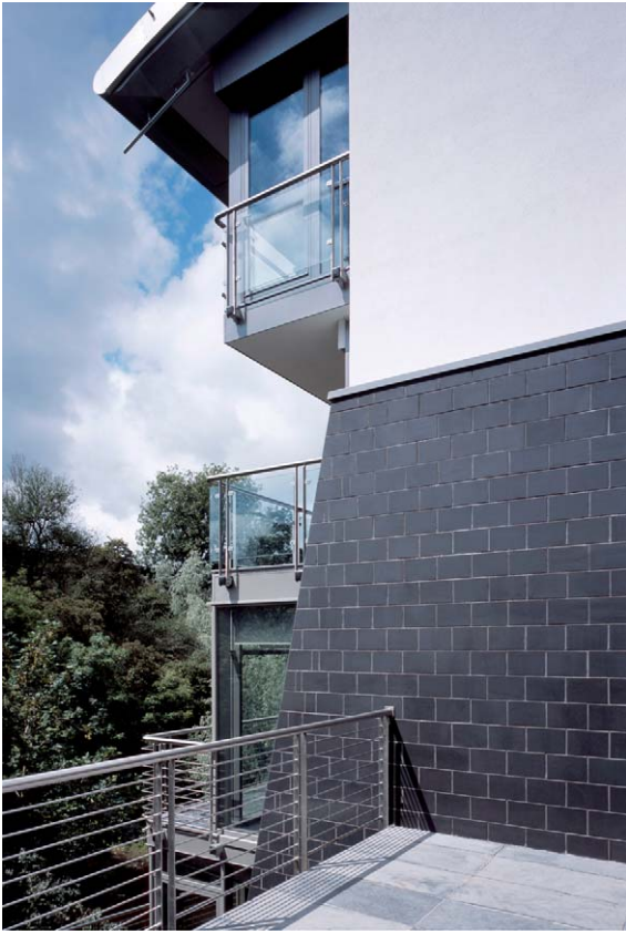
Fig. 2.9 Fairfaced blockwork – IDP Offices, Glasgow. Architect: IDP. Photograph: Courtesy of Ibstock Brick Ltd
