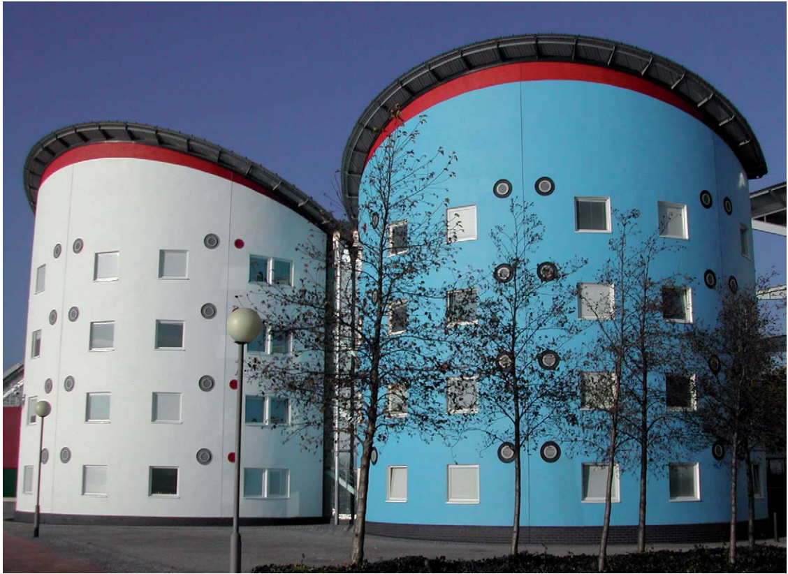
Fig. 3.23 Continued. Rendered blockwork – University of East London, Docklands Campus. Architects: Edward Cullinan Architects. Photograph: Arthur Lyons
