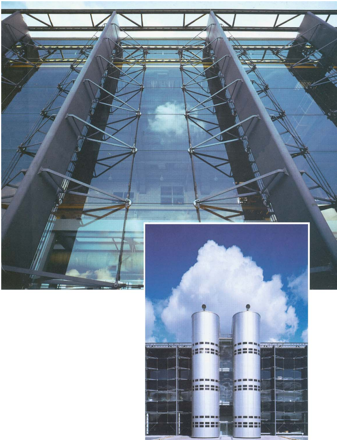
Fig. 7.21 Glazing system – Financial Times, Docklands, London. Architects: Nicholas Grimshaw and Partners. Photographs: Courtesy of Nicholas Grimshaw and Partners, Jo Reid & John Peck
