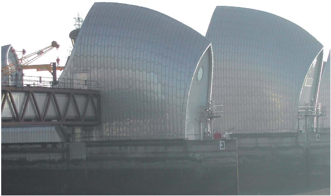
Fig. 4.23 Thames Barrage, London. Photograph: Arthur Lyons
