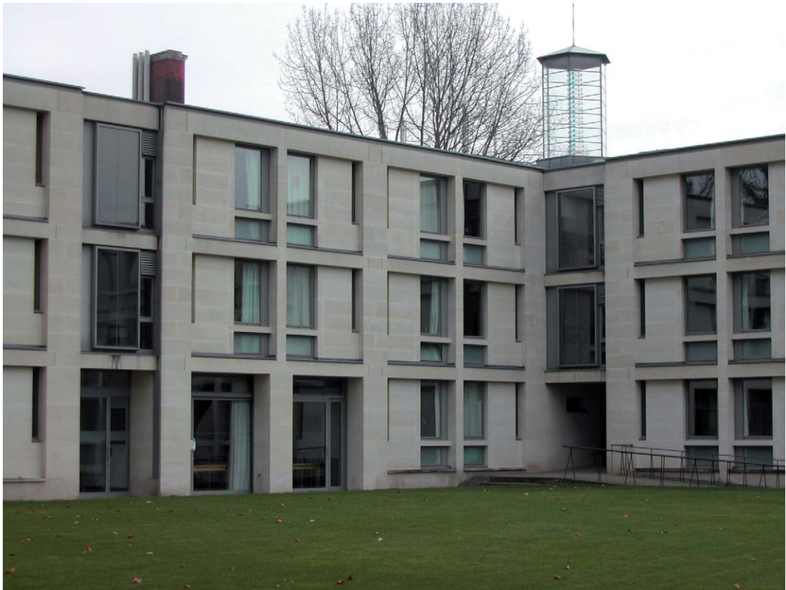
Fig. 9.6 Bath Stone – Foundress Court, Pembroke College, Cambridge. Architects: Eric Parry Architects. Photograph: Arthur Lyons
