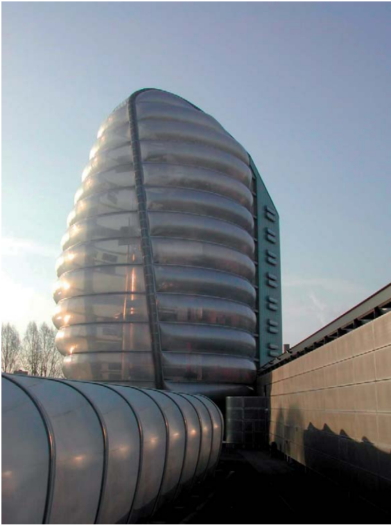
Fig. 10.15 ETFE – National Space Centre, Leicester. Architects: Nicholas Grimshaw and Partners. Photograph: Arthur Lyons
