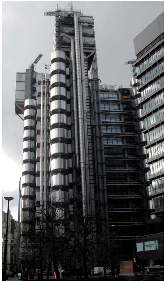
Fig. 5.16 Stainless steel construction – Lloyd's Building, London. Architects: Richard Rogers. Photograph: Arthur Lyons
