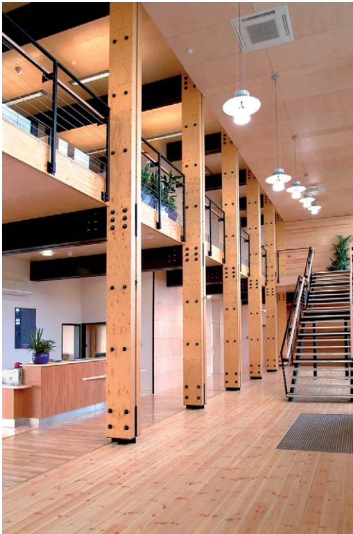
Fig. 4.25 Laminated veneer lumber (LVL) construction – Finnforest Office, Boston, Lincolnshire. Architects: Arosuo and Vapaavuori Oy. Photograph: Courtesy of Finnforest
