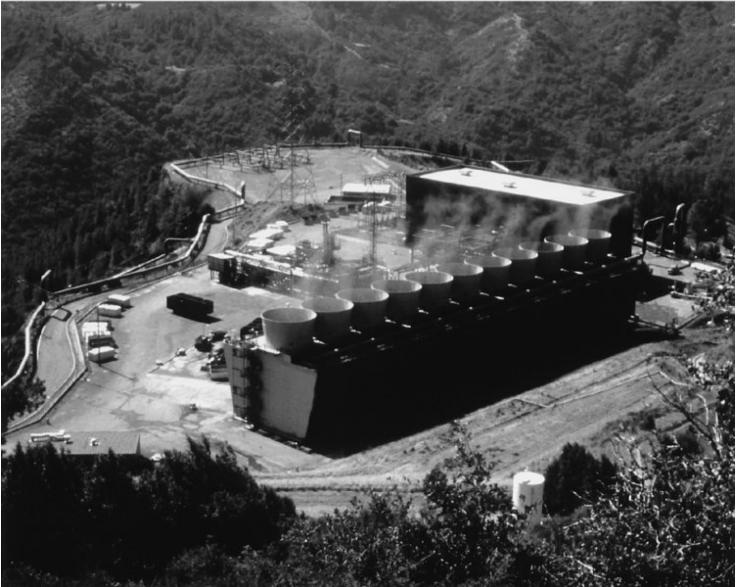
Plate 4.6 Geothermal power plant, California
