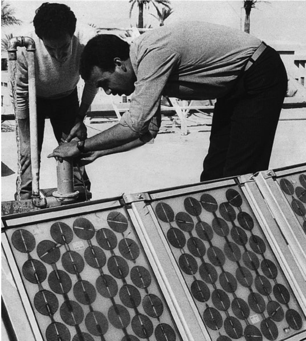
Plate 4.5 Solar energy provides power for a water pump in Morocco
