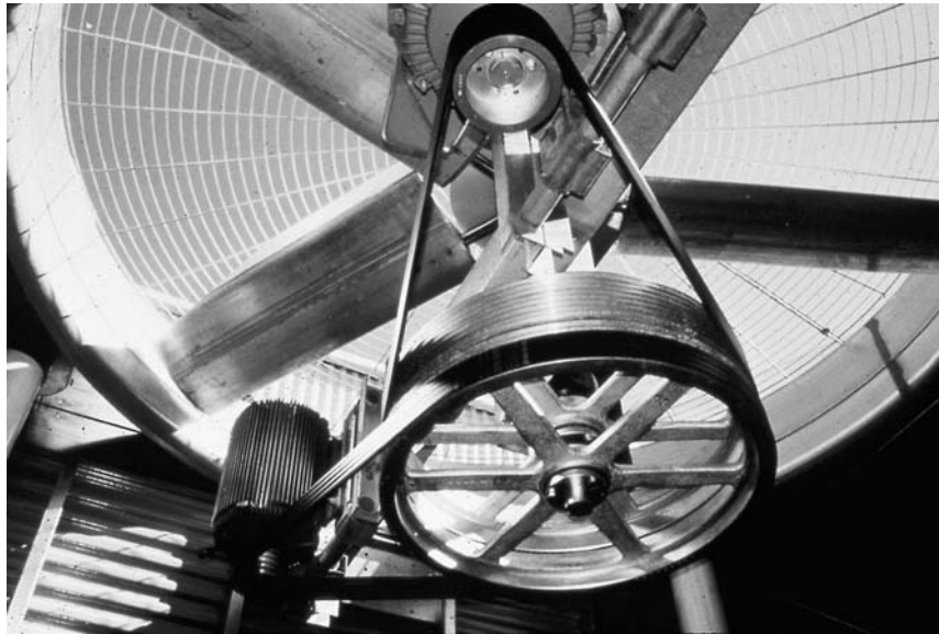
FIGURE 10.8. Typical cooling tower belt drive assembly. (Courtesy of the Baltimore Aircoil Company, Baltimore, Maryland.)
